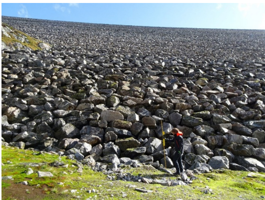
Fig. 1. Placed riprap constructed on Dam Oddatjørn, Suldal, Norway.
