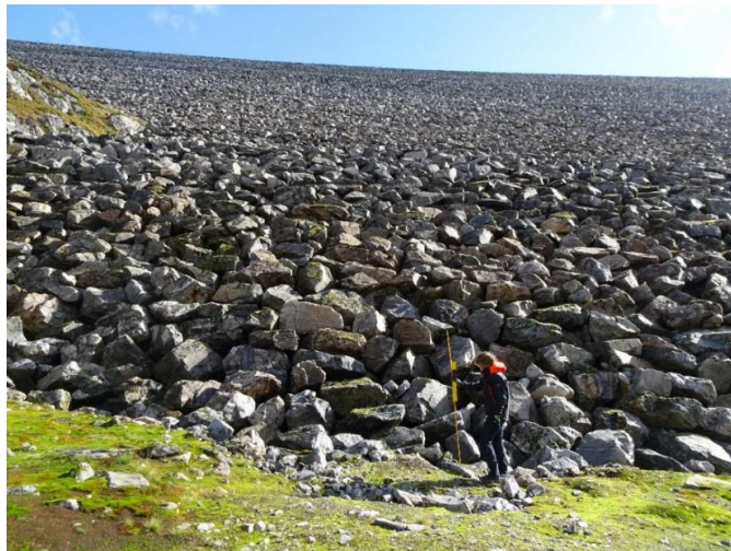
Figure 2. Placed riprap constructed on the downstream slope of dam Oddatjørn, which is a 142 m high rockfill dam constructed in Suldal, Norway (Photo: GHR Ravindra, NTNU).
