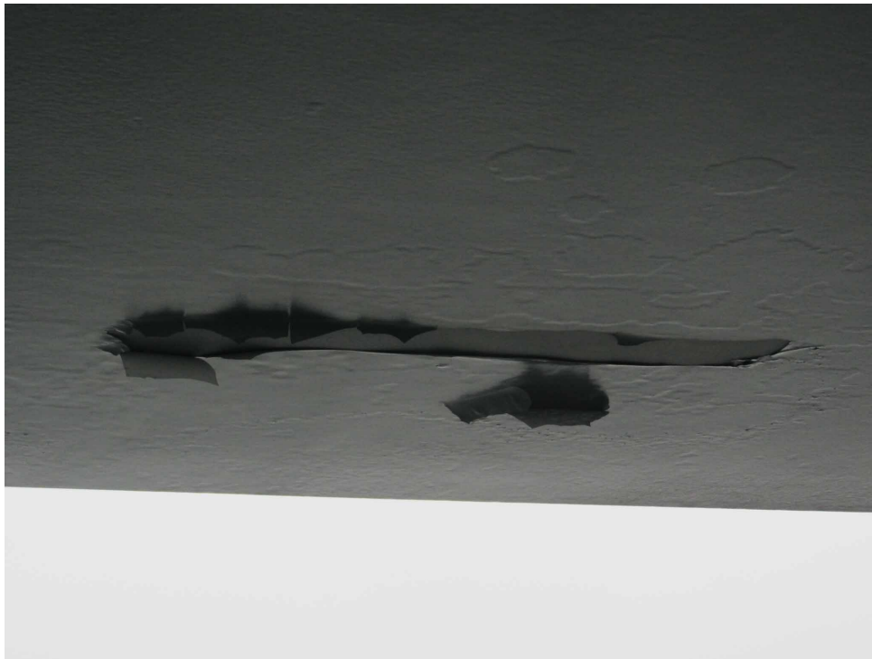
Figure 5.1: Example of the coating (IOZ) on a bridge assessed as good. Few areas of this kind of top coat flaking is accepted
