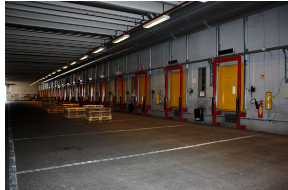
Figure 6: Loading ramps at Nydalen printing facilities
