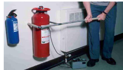
Figure 12: Level gauge used to measure fluid level inside fire extinguishers (IAEA, 2003)
