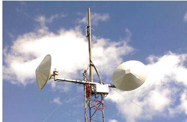
Figure 37: Example of Radio Link with sender and receiver (RadioLink Telemark AS, 2014)
