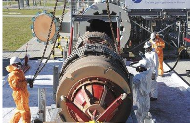
Figure 34: The removal of a pipeline pig (Source: http://www.nord-stream.com/press-info/images/arrival-of-the-inline-inspection-tool-in-lubmin-3502/ )
