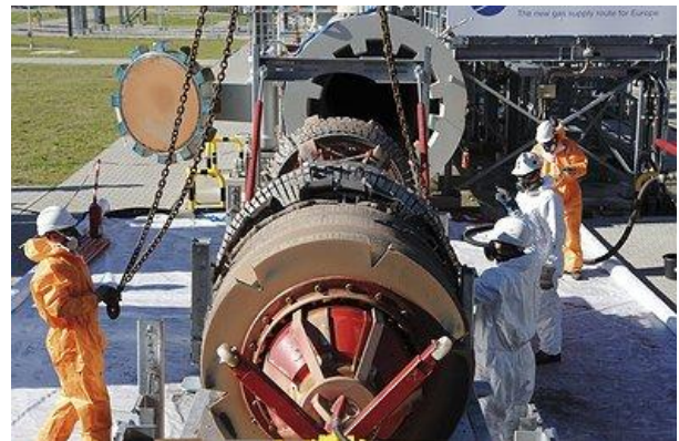
Figure 23: The removal of a pipeline pig (Source: http://www.nord-stream.com/press-info/images/arrival-of-the-inline-inspection-tool-in-lubmin-3502/ )
