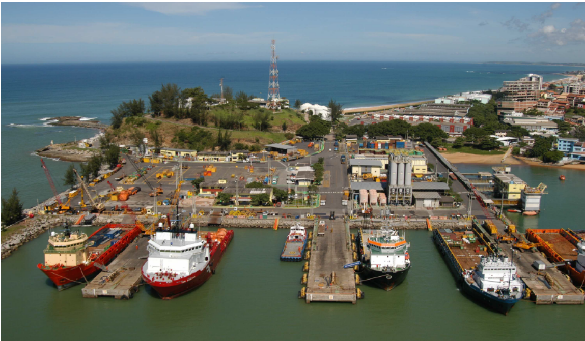
Figure 1.5: Terminal Alfandegado de Imbetiba (TAI)
