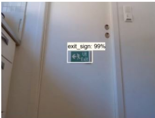
Figure 5.10: Exit sign result
