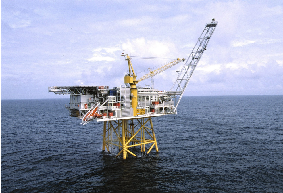
Figure 1.6: Huldra. A fixed platform. Photo: Kjetil Alsvik/Statoil
