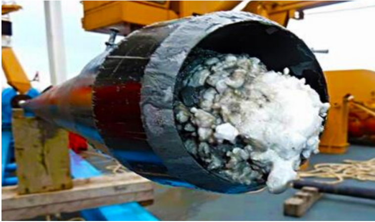
Figure 2.7: Hydrates plugging a flowline on a gas producing well (Jozian and Vafajoo, 2018)
