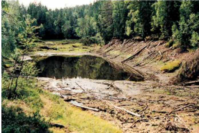
Figure 4.4: Photo by L. Erikstad of Puttjern above the Romeriksporten railway tunnel. Puttjern was a water source to the high inflows in the tunnel, and the water table consequently got drained (Kveen and Lindstrøm, 2005).
