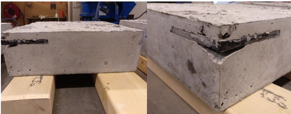
FIGURE 46: LATERAL VIEW AND DETAILED VIEW OF THE 15MM DEPTH SLAB
