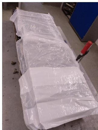
FIGURE 44: CONCRETE SLABS COVERED WITH PLASTIC FOR CURING
