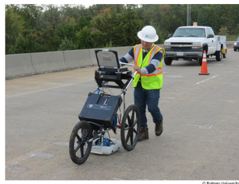
FIGURE 16: DATA ACQUISITION ON A BRIDGE DECK USING GROUND- COUPLED GPR [15]
