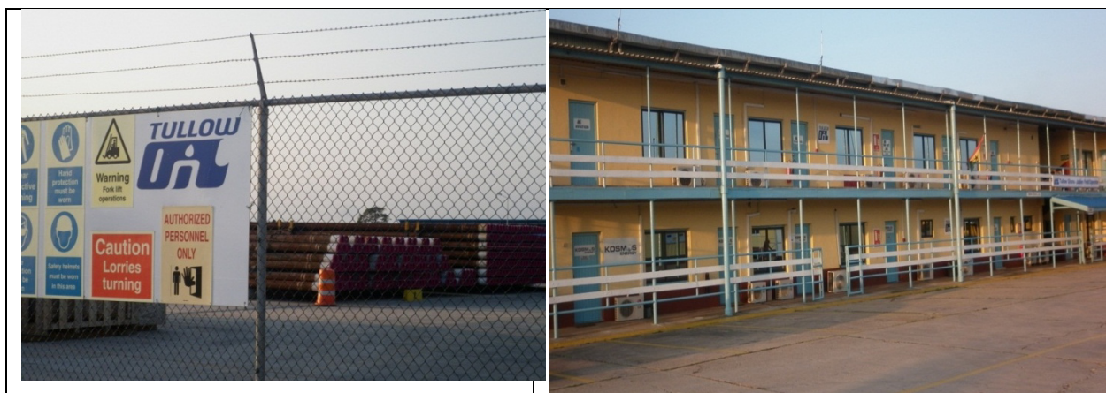
Protected storage area for oil pipes
