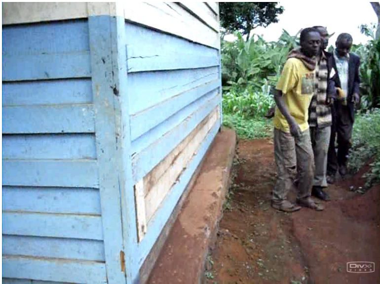
Figure 5: Photo showing timber as building material
