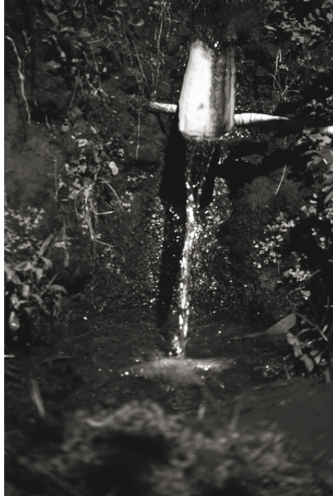
Fig. A3:2: Domestic drawing point on a secondary branch. Photograph by author.
