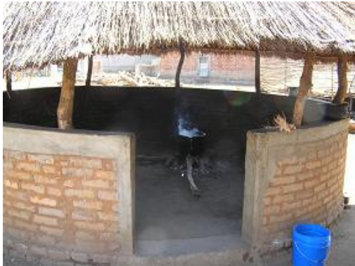
Figure 17 Fireplace at the Sister's camp of the Anglican Church in Masasi
