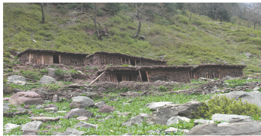
Fig.12. A high altitude wood and mud-built settlement in the Village of Bheri.
