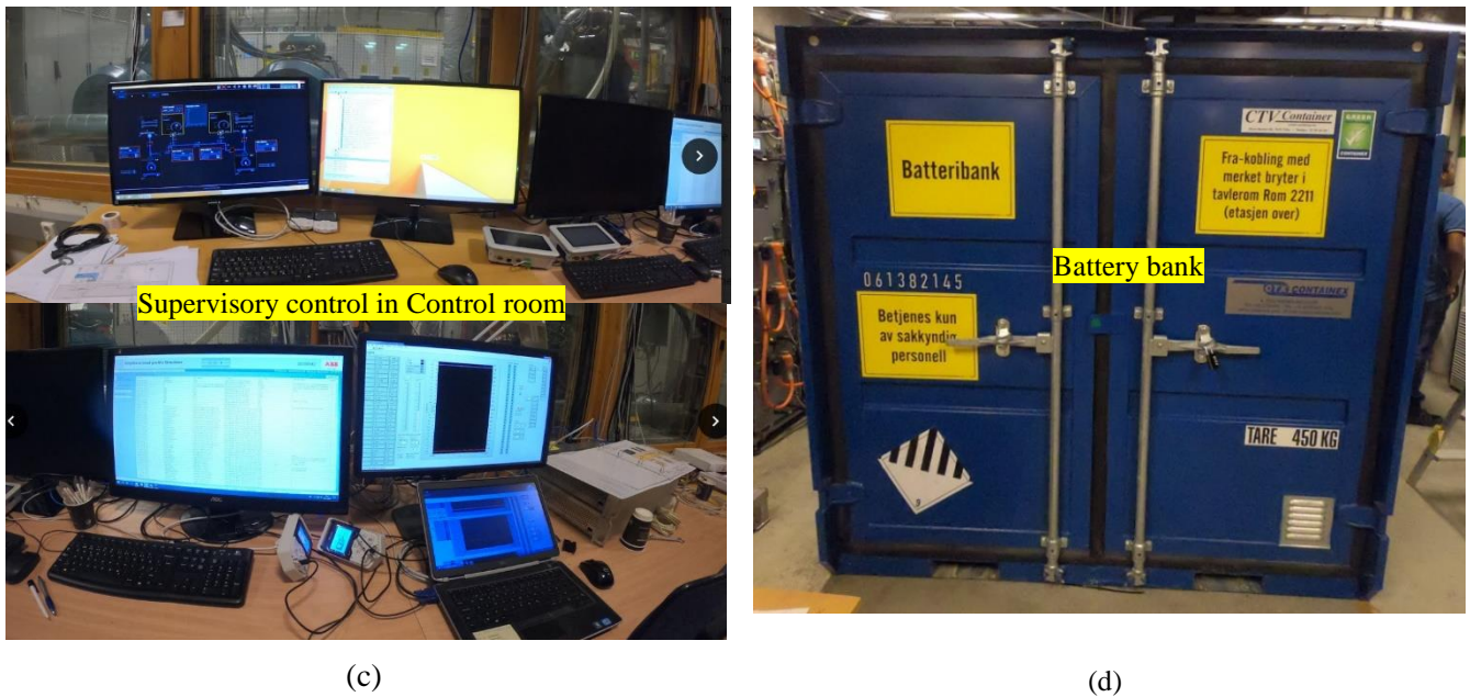
Figure 4 (a) Variable Speed Diesel Engine – Generator Sets, (b) Electric loads, (c) control room and (d) battery bank.
