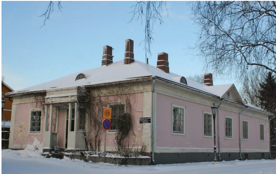
Figure 158. The plastered notched log construction – a legacy of a new trend of Classicism as a counter-reaction to the emerging Swiss Chalet Style and other diverse historical styles at the beginning of the 20th century (Photo by Giedrė Jarulaitienė, 2008).
