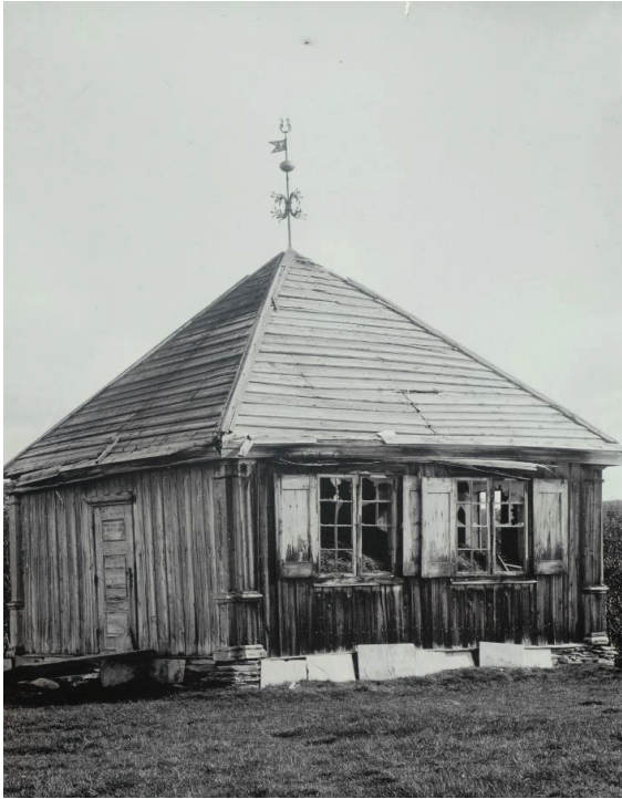
Figure 24. The neglected Baroque garden pavilion ( lysthus ) reused as a hay barn. (Photographer and date unknown, Gunnerus - Spesialsamlinger ved NTNU Universitetsbiblioteket, VI-Uf-72721)
