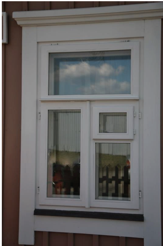
Figure 254. Such details of traditional craftsmanship as the separate air vents were considered as important components of the reconstructed building not only by the architect, but the owner as well (Photo taken by Giedre Jarulaitiene, 2017).
