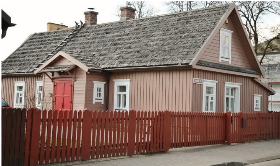
Figure 253. The façades of the reconstructed building were historized not only by following the architectural forms, typical of the Minor Town, but also by using such traditional materials on the exterior as wooden boarding and wooden roofing (Photo taken by Giedre Jarulaitiene, 2017).
