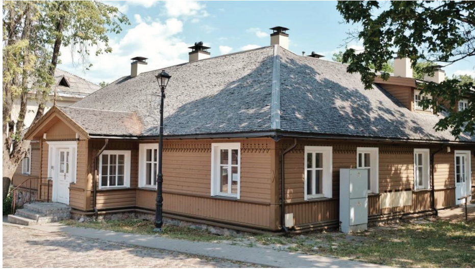
Figure 233. One of the few reconstructed buildings, which was rebuilt by using the notched-log building technique and historized external embellishments (Photo taken by Giedrė Jarulaitienė, 2019).
