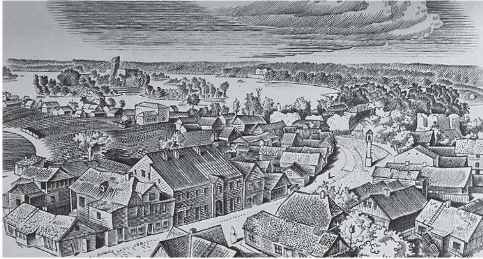
Figure 215. The central townscape of Trakai captured before the outbreak of World War II (The drawing by W. Romanowicz. Archives of The Department of Cultural Heritage under the Ministry of Culture. F. 11, I. 5, f. 162, p. 100).
