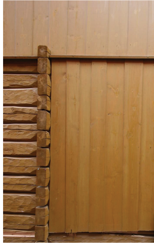
Figure 128. The copy of panelling, produced in the “procedurally authentic” way (Photo taken by Giedrė Jarulaitienė, 2011).
