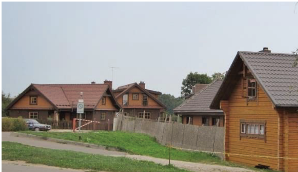
Figure 245. During the last decades of urban conservation, a paradox emerged in the Old Town of Trakai – modern, but historized, masonry constructions were constantly covered up by wooden panel cladding (Photo taken by Giedrė Jarulaitienė).
