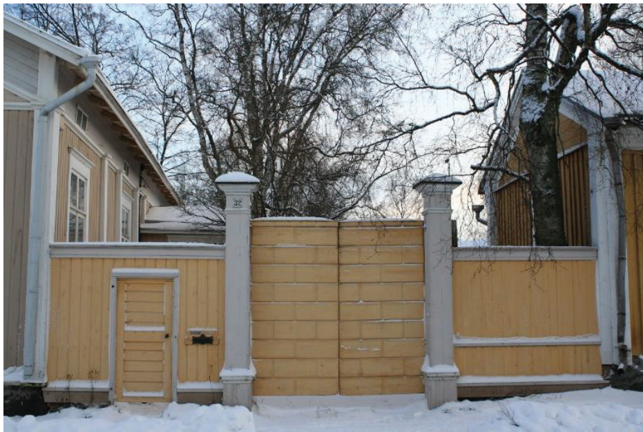
Figure 154. The image of ashlar masonry applied to wooden architectural details (Photo taken by Giedrė Jarulaitienė, 2008).
