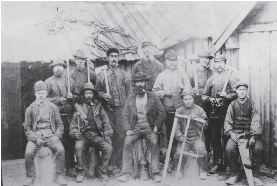
Figure 32. A group of craftsmen with their hand tools. (Photo taken by Iver Olsen, date unknown; ©Rørosmuseet, RMUB.251135)
