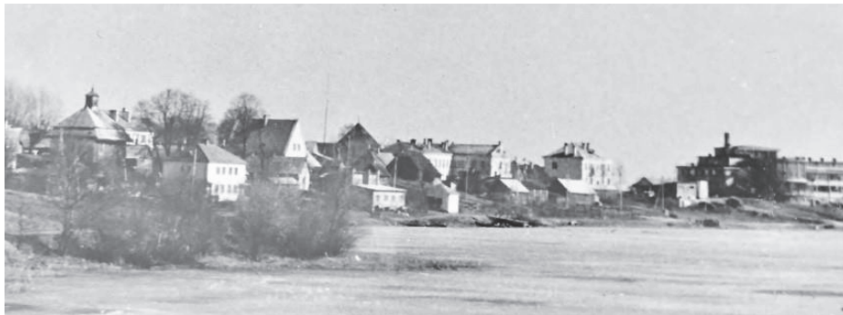
Figure 218. The dissonances in the townscape of Trakai, brought by modernistic buildings, were subsequently used as an argument for initiating the urban conservation in Trakai (Photo taken by Stanislovas Mikulionis, 1964. Vilnius Regional State Archives, F1019, F. 12, f. 19582).
