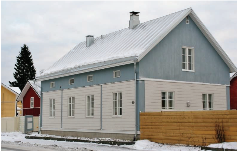
Figure 179. The example of increasing adjustments of modern infill architecture by following the scale, forms and façades of historical buildings from the 19th century. The expressive details, such as restrained corner and frontal “pilasters”, were contrarywise indrawn and in that way the actual recency of the building’s design and construction was displayed. (Photo taken by Giedrė Jarulaitienė, 2008).
