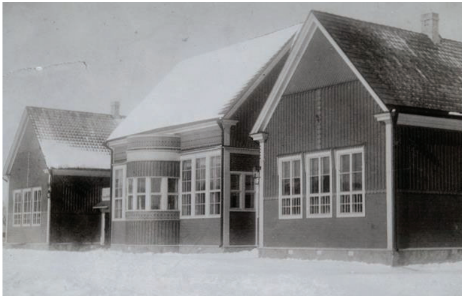
Figure 164. The main façade of K. H. Renlunds elementary school, designed by architects Ivar and Valter Thomé in 1907 and built in the new wooden urban area of Kokkola. “All the walls are built from upright, dried pine wood. That enabled to cover the walls without disruptions with wooden clapboards externally and wallpaper or painting internally. [...] Gamlakarleby must be congratulated that elementary school children will learn in modern and well-furnished facilities. That will certainly influence the progress of all the people, who will visit the school”(Thomé V., 1909, p. 115). (National Board of Antiquities, HK19590916:2).
