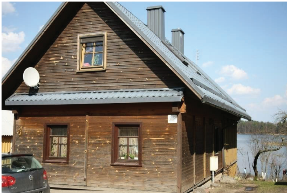
Figure 234. Even though one of the oldest residential buildings from the end of the 18th century in the Minor Town (Tarnauskienė, 1998b, 80) was renovated by using traditional materials and new windows, divided according to their historical prototypes, the modern modus operandum used in the reproduction of these new building elements was obvious (Photo taken by Giedrė Jarulaitienė, 2017).
