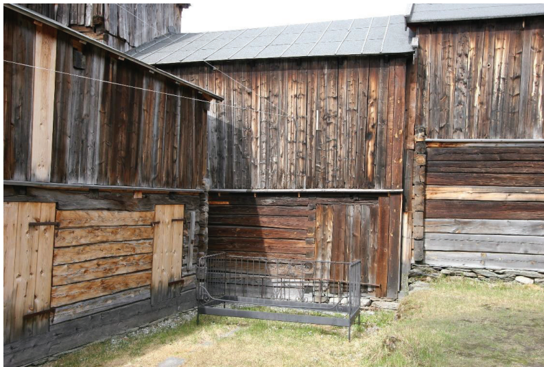
Figure 72. The overall image of the inner yard of Per Amundsagården, “disturbed” by the bit-by-bit replacements of the decayed parts (Photo taken by Giedrė Jarulaitienė, 2011).
