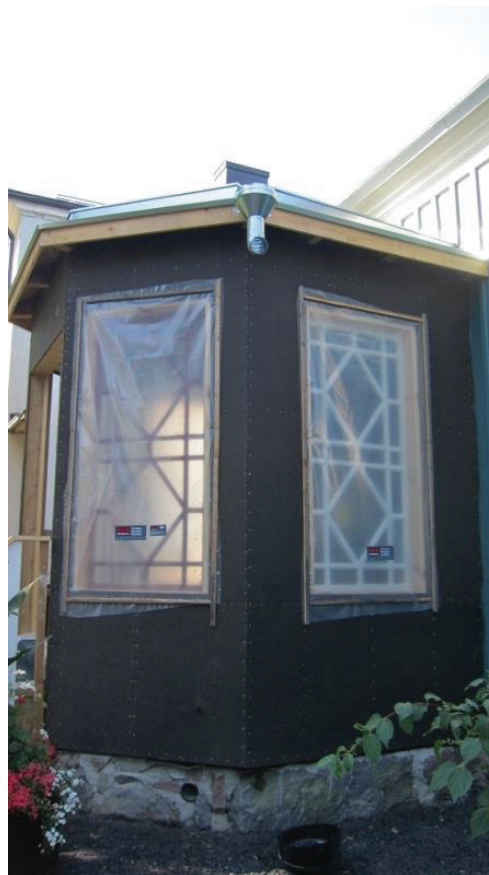
Figure 189. The old windows from the old rectory were re-used in the renovation of Knape's house. (Picture taken by Giedrė Jarulaitienė, 2011)
