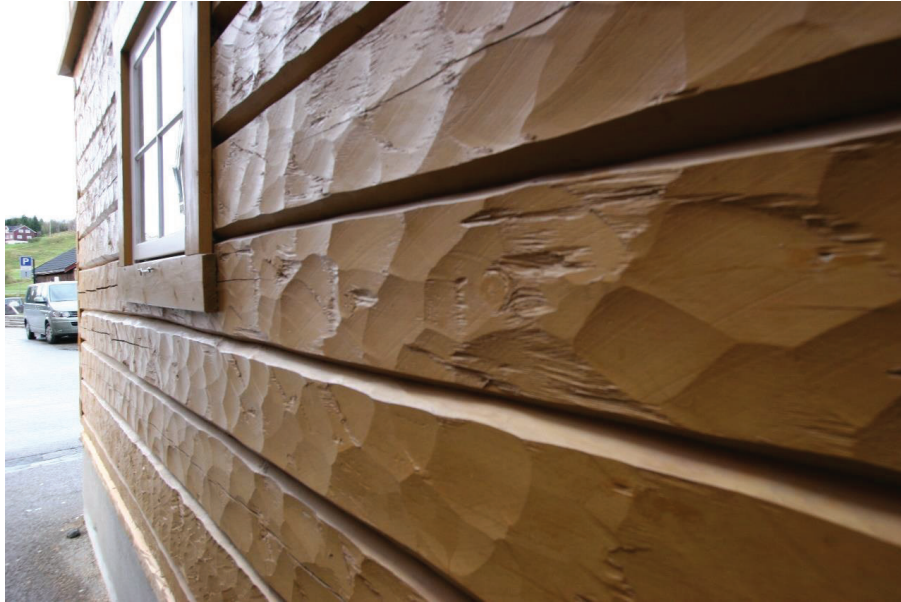
Figure 120. The external side of sawn logs was also manually hewn to demonstrate the high quality of carpentry (Photo taken by Giedrė Jarulaitienė, 2011).
