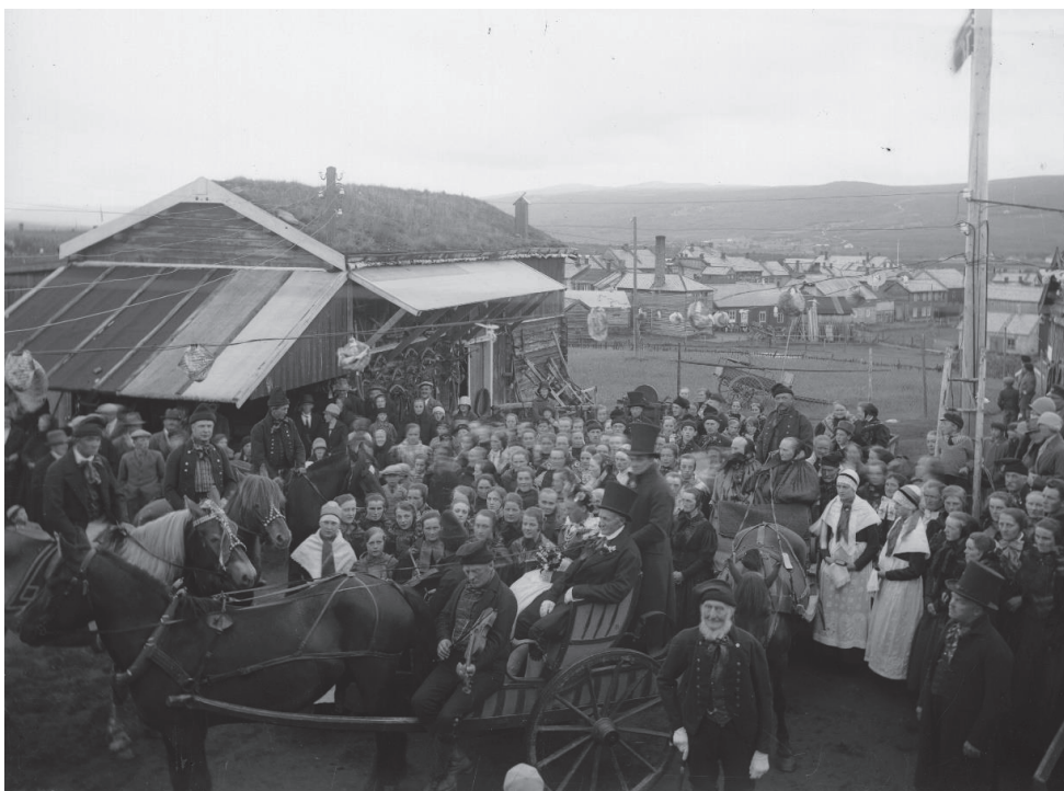
Figure 19. The theatrical parade at the opening ceremony of the exhibition at Aasengården. (Photo taken by Iver Olsen, 1930; ©Rørosmuseet RMUB.251840)
