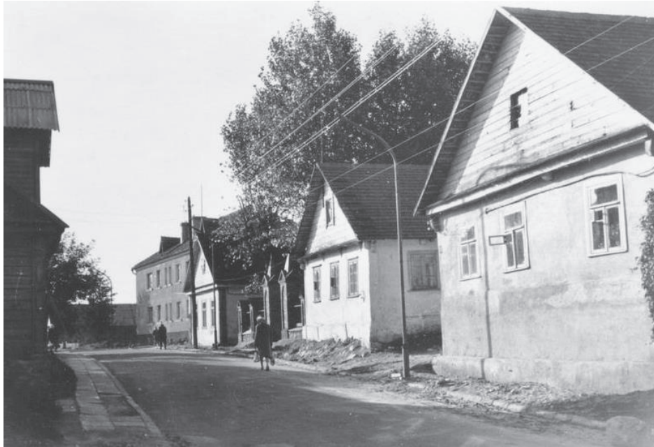
Figure 244. The plastered façades of log buildings dominated the Karaitė Street in the Minor Town of the Old Town of Trakai (Photographer unknown, 1963. Trakai History Museum, TIM GEK 11789/1)
