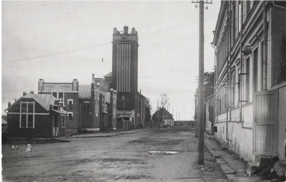
Figure 162. The outstanding power plant in Jugend style, designed by architects Gustaf Strengell and Sigurd Frosterus. Built in 1906, next to Neristan in Kokkola (Photo taken in 1920, National Board of Antiquities, HK19571229)
