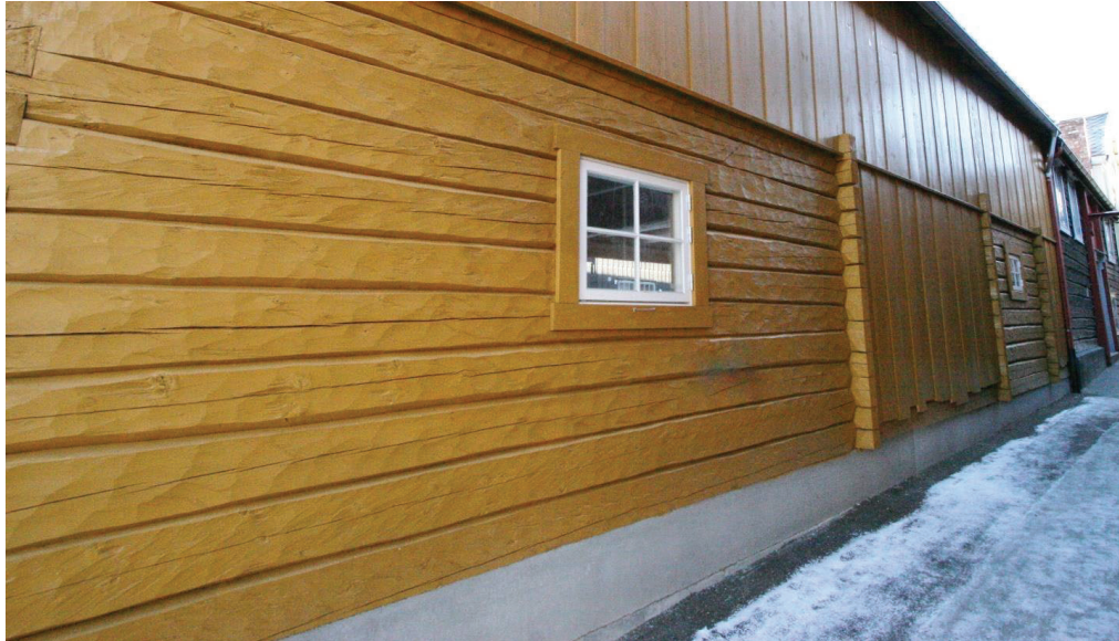
Figure 132. The aesthetic discrepancy between the smooth and straight concrete foundations vs. rough and variable surfaces with traces of manual woodworking (Photo by Giedrė Jarulaitienė, 2009).
