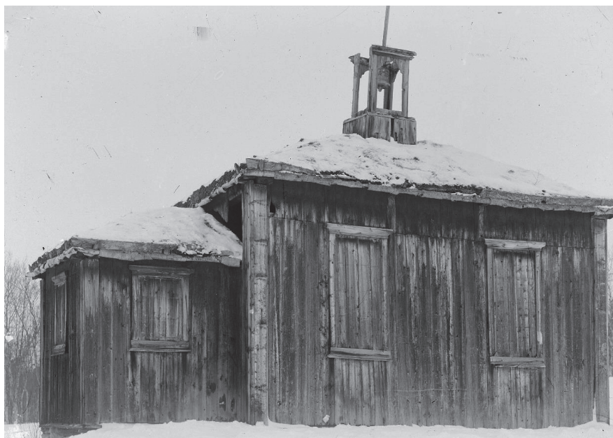
Figure 26. The exceptional form of Engan garden pavilion, called “P. P. Hiort’s church”. (Photo taken by Iver Olsen. ©Rørosmusset RMUB.251118)
