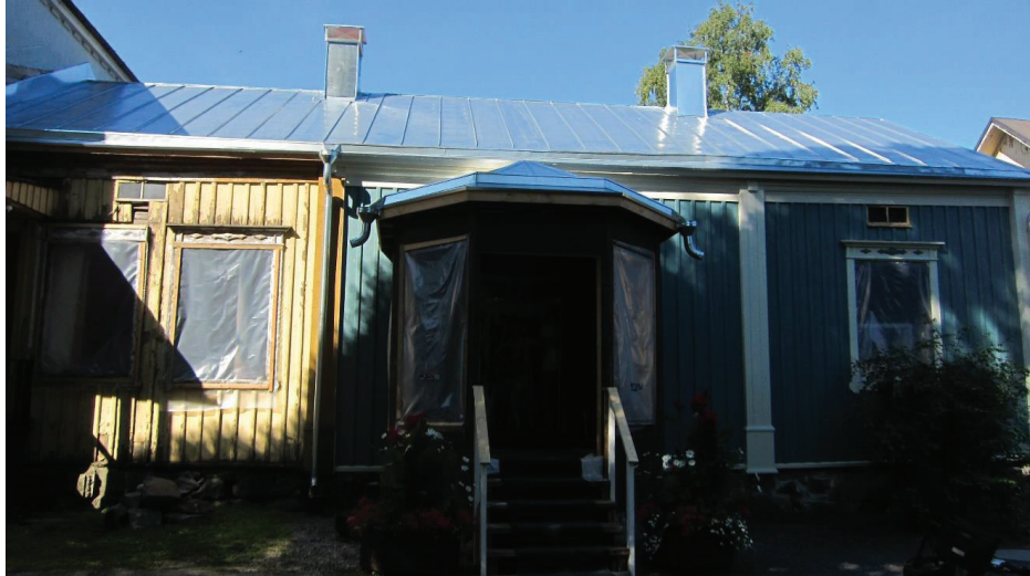
Figures 190, 191. The creative adaptation of recycled windows in a newly-replaced porch on the back façade of the Knape's house. (Pictures taken by Giedrė Jarulaitienė, 2010, 2011).
