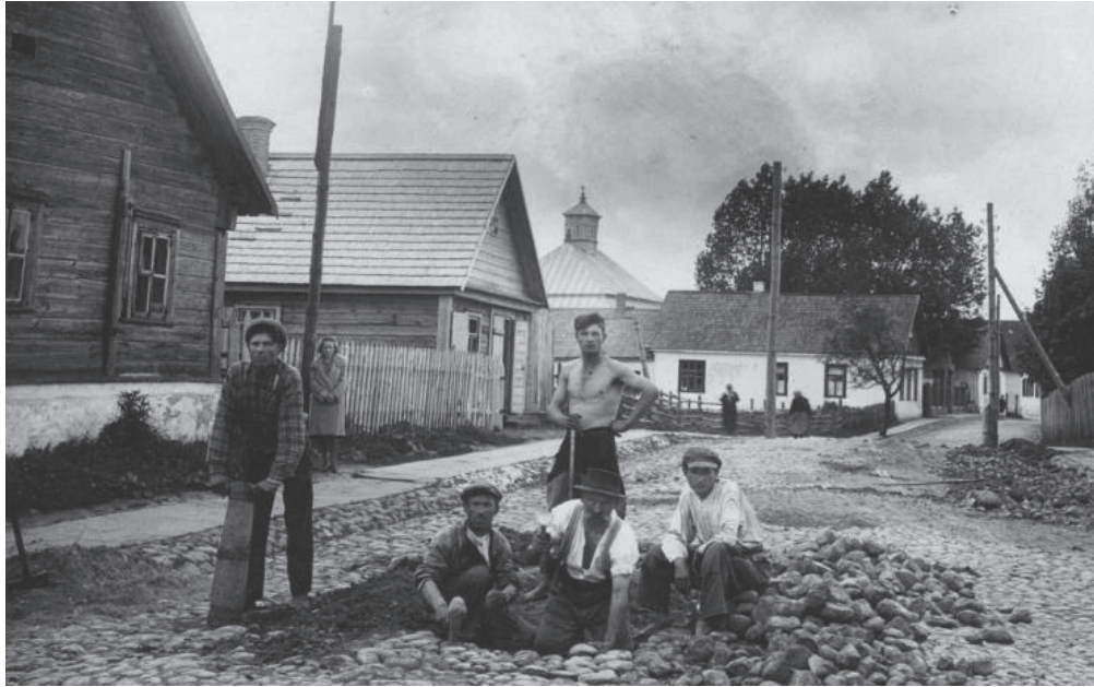
Figure 246. The second house on the left side – the original notched-log construction, dated to 1930. The original roof was covered with wooden shingles (Photographer unknown, 1932. Trakai History Museum).
