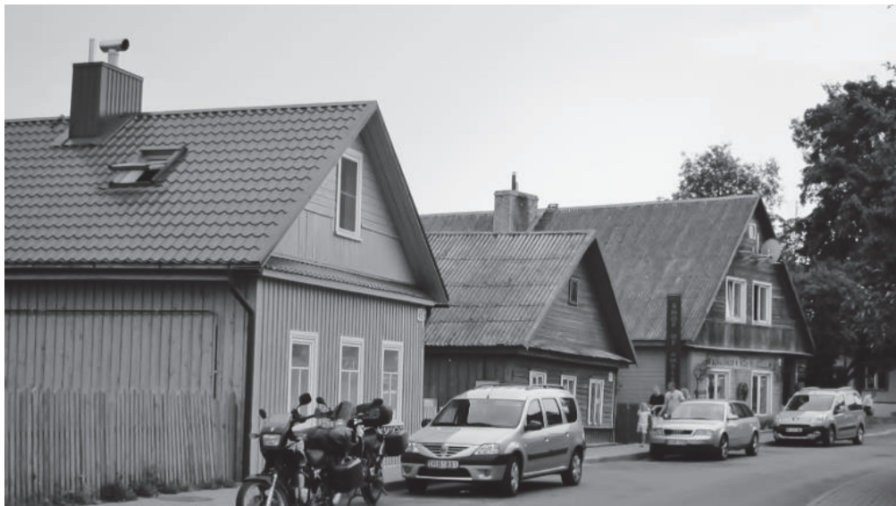
Figure 230. The first building on the right side is the same building, which was covered with wooden roofing as the above-presented historical picture depicted. The wooden roofing was changed for the imitation of clay tiles, while the fireproof asbestos slates from the soviet period were sustained (Photo taken by Giedrė Jarulaitienė, 2010).
