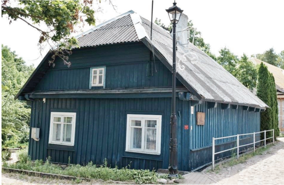
Figure 207. Figure 207. The building from the 1810's – 1820's was used as a parish school, which was patronized by Vilnius University in 1803-1830. The present asbestos slate roofing hides the original roofing of wooden shingles beneath. (Photo taken by Giedrė Jarulaitienė, 2019).
