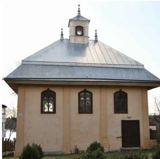
Figure 209. The plastered log house of prayer was decorated with a tower in 1894 (Photo taken by Giedrė Jarulaitienė, 2010).
