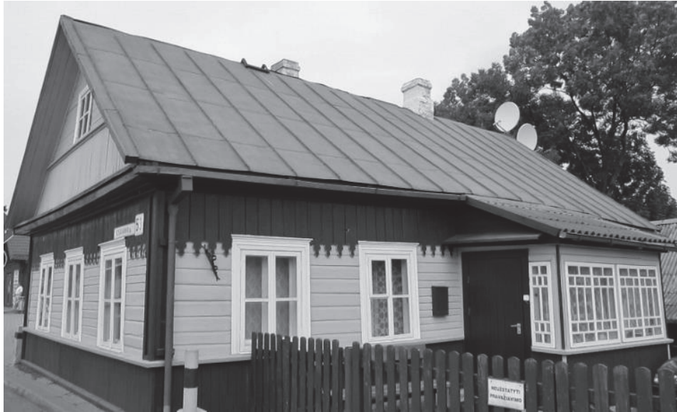
Figure 229. The tin-plate roofing was sustained throughout the soviet period of urban conservation in the Minor Town of Trakai (Photo taken by Giedrė Jarulaitienė, 2010).
