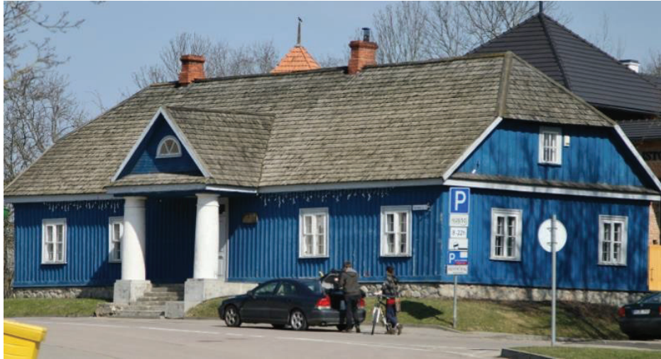
Figure 208. The former Imperial Post Office sustained some of its original architectural forms, typical of the beginning of the 19 th century (i.e. half-hip roof), despite the continuous functional and architectural transformations throughout the turbulent history of the town (Photo taken by Giedrė Jarulaitienė, 2017).
