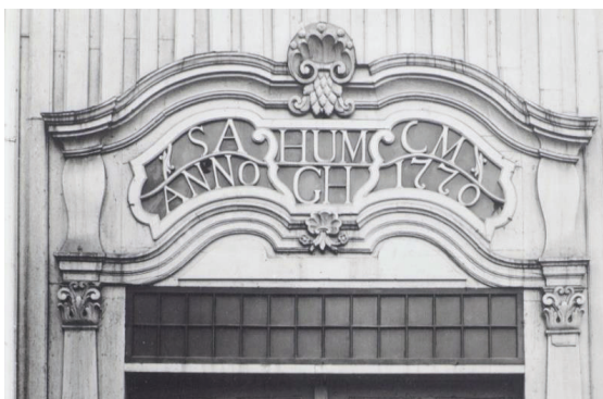
Figure 45. The appropriate implementation of Rococo in wooden architecture was a distinct trøndisk feature, according to H. Vreim. However, Harmonien in Trondheim was probably designed by H. Kühnemann or Johan Daniel Berlin from Memel. (Bratberg, T. V., 2008, p. 222; Kavli, G., 1966, p. 309). The entrance portal to Harmonien was claimed to be H. Kühnemann’s exceptional piece of fantasy, which “hardly is a common local joiner’s work” (Kavli, 1966, 310). (Photographer unknown, 1913, Gunnerus - Spesialsamlinger ved NTNU Universitetsbiblioteket, UBT-TO-075281_01_1)
