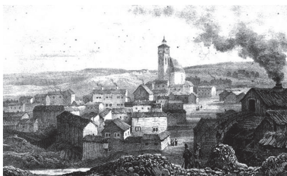
Figure 49. The workshops of smiths, joiners, fire bellow makers and wheelwrights, belonging to the Røros Copper Works at Kurantgården (Lithography, Twining, 1836, 274-275).
