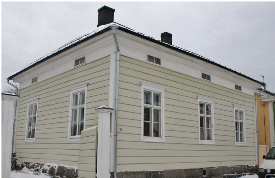
Figure 156. An exemplary model of adaptation of Empire style in a wooden building supplemented with a preferable hip roof (Photo taken by Giedrė Jarulaitienė, 2008).
