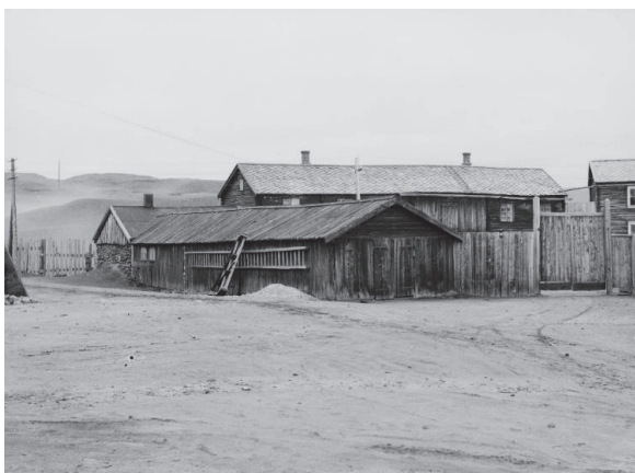
Figure 50. The entrance to Kurantgården where the Røros Copper Works still had its office and workshops. Photo taken before the new mechanical workshops were built in 1940. (Photo taken by Iver Olsen, 1940, ©Rørosmuseet, RMUB.255837)
