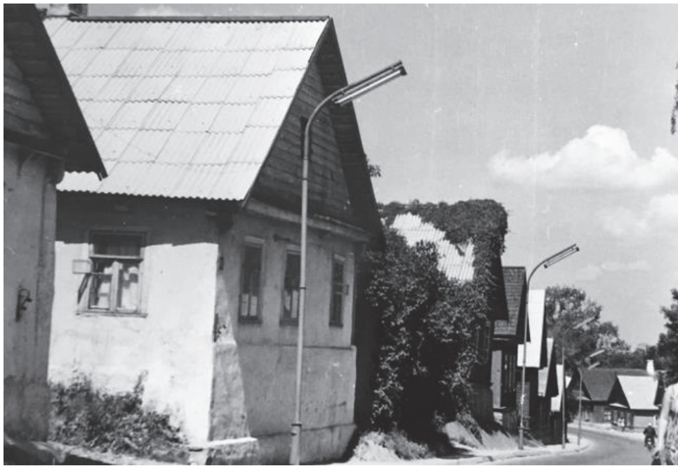
Figure 241, 242, 243. The tradition of concealing log buildings with plaster in order to imitate masonry buildings was common in the Old Town of Trakai throughout history (Photos taken by M. Sakalauskas, 1969. Vilnius Regional State Archives, F. 1019, I. 12, f. 19582).
