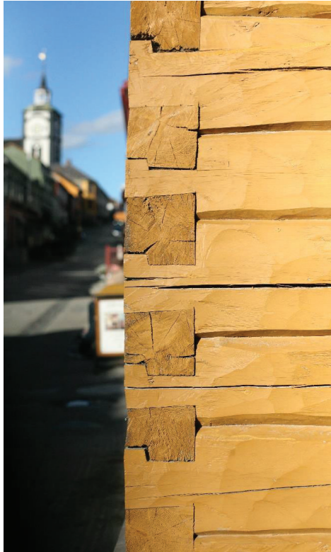
Figure 123. Tooth-edge joints (kamlaft) (Photo by Giedrė Jarulaitienė, 2016).
