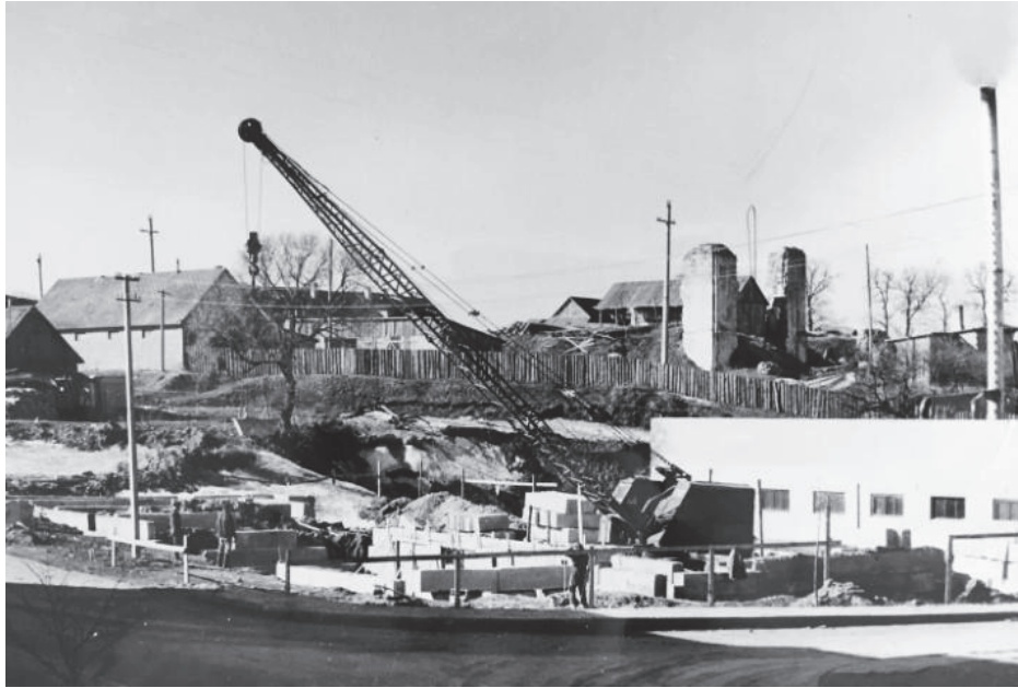
Figure 219. The large-scale constructions next to the ruins of the complex of the Bernardine Monastery (Photo taken by Stanislovas Mikulionis, 1964. Vilnius Regional State Archives, F1019, F. 12, f. 19582).
