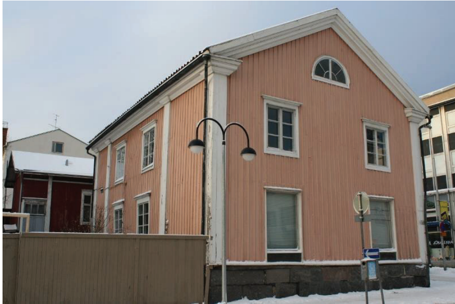
Figure 148. A two-storey building, constructed by the above-mentioned Donners family of local merchants in 1810, manifested the masonry principles of Neo-Classicism in wooden constructions (Photo taken by Giedrė Jarulaitienė, 2008).
