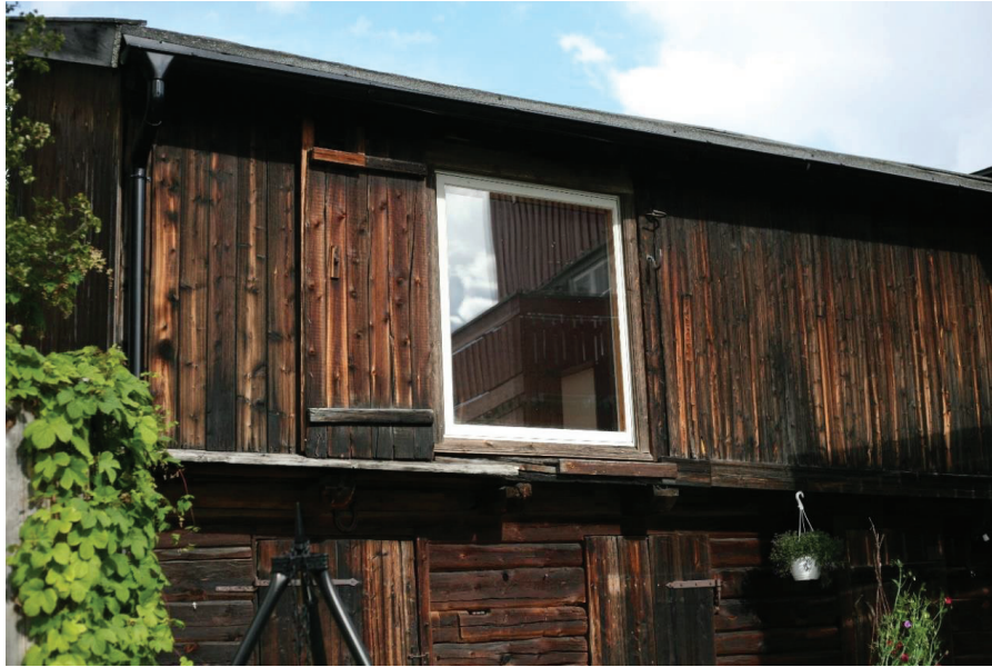
Figure 61. The choice for contemporary windows clearly stating their date of origin, instead of copies of historical windows, is getting more popular in the old town centre of Røros (Photo taken by Giedrė Jarulaitienė, 2016).
