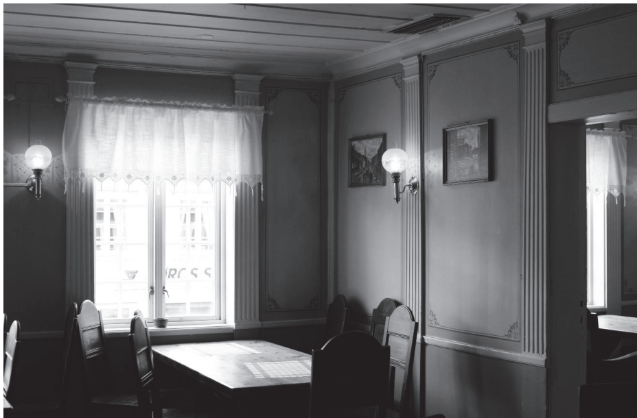
Figure 96. Pilasters – the main decorative features of dining room interiors – at Kaffestuggu preserved until today (Photo taken by Giedrė Jarulaitienė, 2016).
