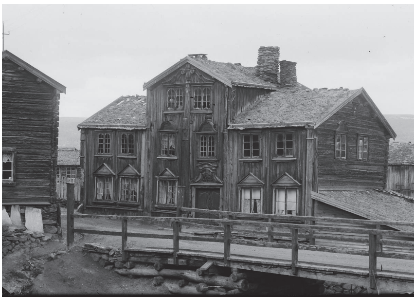
Figure 16. Differing kind of windows and their embellishments testify the reuse of various building materials from other, older buildings. (Photo taken by Iver Olsen; date unknown, ©Rørosmuseet RMUB.251032).
