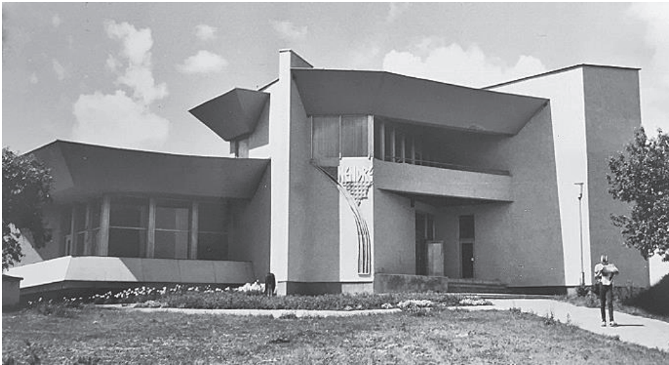
Figure 225. The soviet buildings fell into Zone F or were approved to be modified as in the case of the restaurant “Nendrė” (Photo taken by Giedrė Jarulaitienė, 2017).
