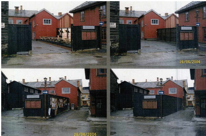
Figure 103. The planked fence, surrounding the backyard of Kaffestuggu. (Photographer unknown, 2004, The private archive of Bergstadens Vel).
