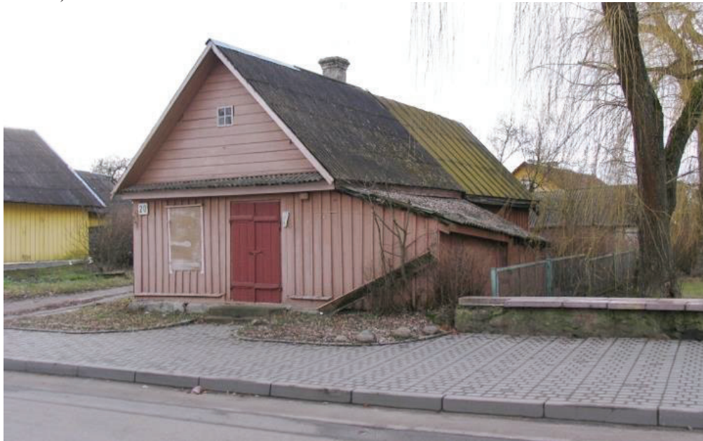
Figure 247. The original Karaite dwelling as documented before the demolition (Photo taken by Dainius Labeckis, 2007?).
