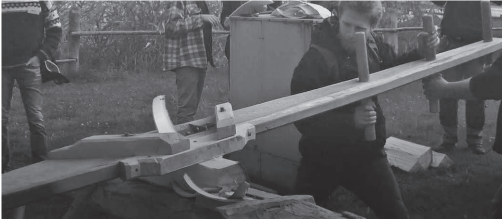
Figure 256. The manual slicing of shingles at the restoration workshop (Photo taken by Giedrė Jarulaitienė, 2015).
