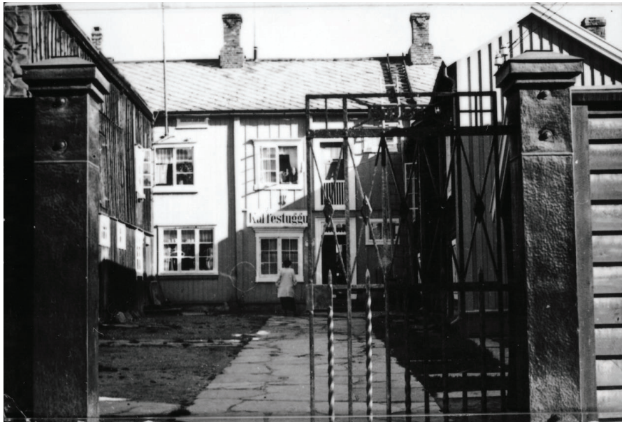
Figure 93. The backyard of Kaffestuggugård, with a newly-planked fence and a copper gate installed. The outbuilding is already missing, but the back side of the main building was still unchanged at that time. (Photographer unknown, 1936-1938 (?), ©Rørosmuseet).
