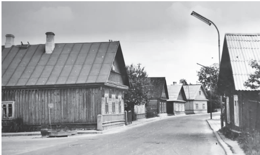
Figure 228. The streetscape of Karaites' Street in the Minor Town of Trakai. The first building on the left side of the street is documented to be covered with tin-plate roofing, while the third one was still covered with wooden roofing (Photo taken by M. Sakalauskas, 1969. Vilnius Regional State Archives, F. 1019, I. 12, f. 19582).
