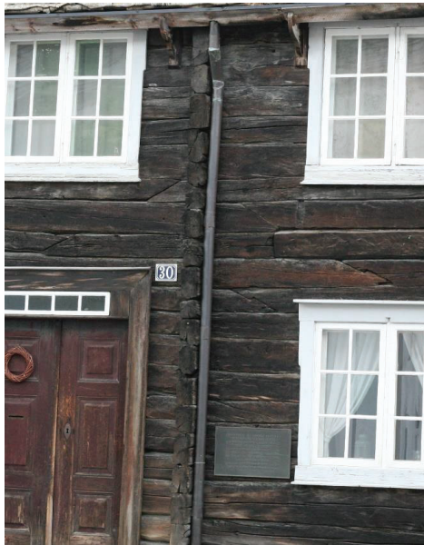
Figure 70. The traces of splicing new log elements at Per Amundsagården (Photo taken by Giedrė Jarulaitienė, 2016).
