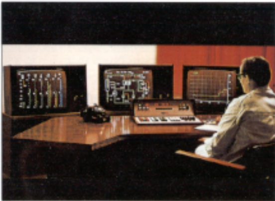
Figure 4. The OPCOM system that for six weeks in 1972 controlled the Halden Boiling Water Reactor
