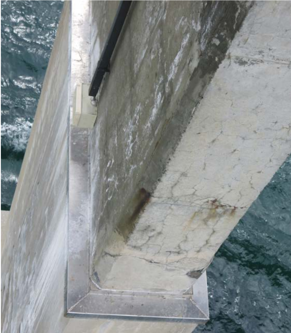
Figure 5-4 Northern side of pillar 17
