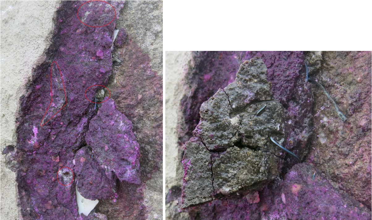
Figure 5-3 Highlighted acidic areas of the mortar from the freshly broken surface.
