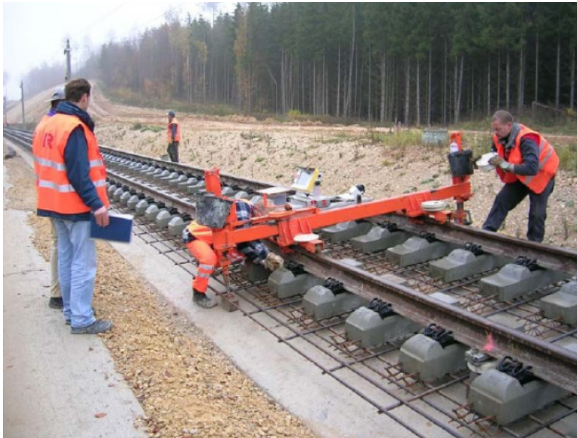
Figure 31 Installation of Rheda 2000 system at high-speed line Nuremberg-Ingolstadt. Top-down construction (Lechner, 2007).
