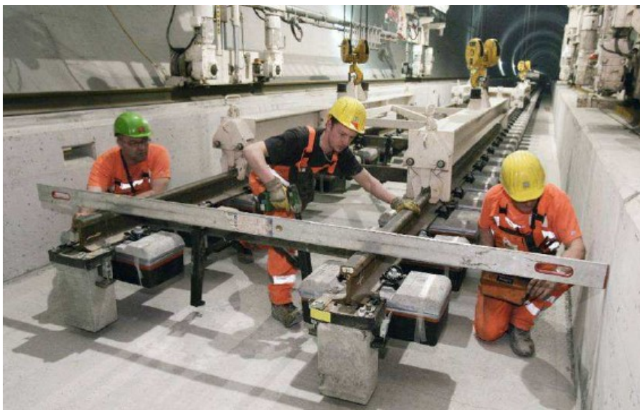
Figure 46 Installation of LVT by Rhomberg Bahntechnik AG (Sonneville AG, 2011)
