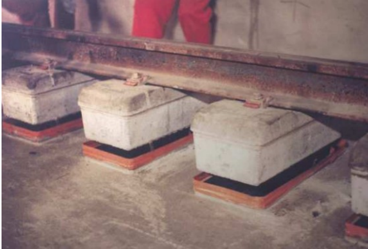
Figure 49 Lifted LVT supports (Sonneville AG, 2019a)
