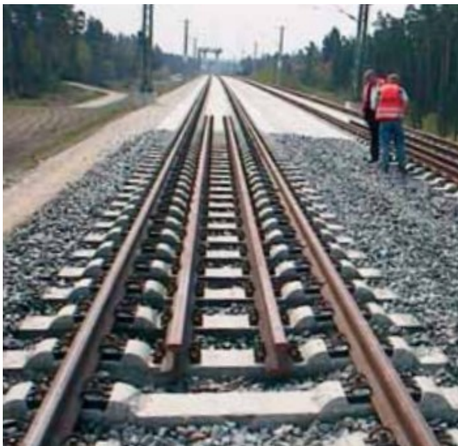
Figure 69 Picture of transition zone for the Rheda 2000 system (RAIL.ONE GmbH 2018)
