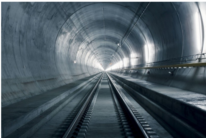
Figure 38 The LVT System in Gotthard Base tunnel (SBB, 2019)
