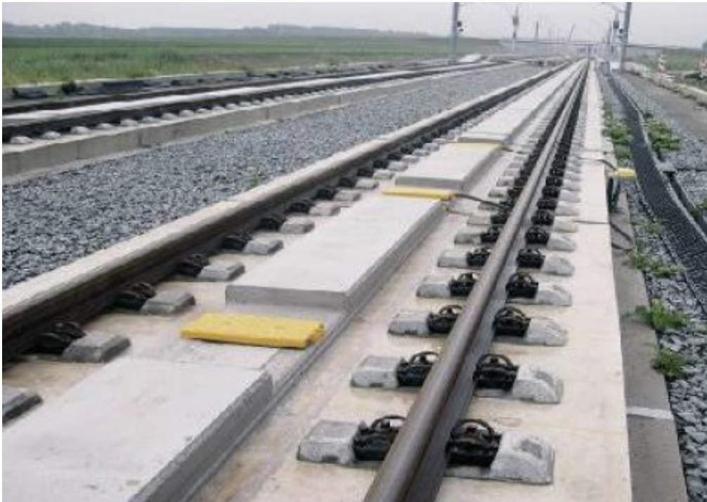
Figure 64 Derailment equipment Rheda 2000 on the HSL Zuid line (von Glasenapp, 2019)
