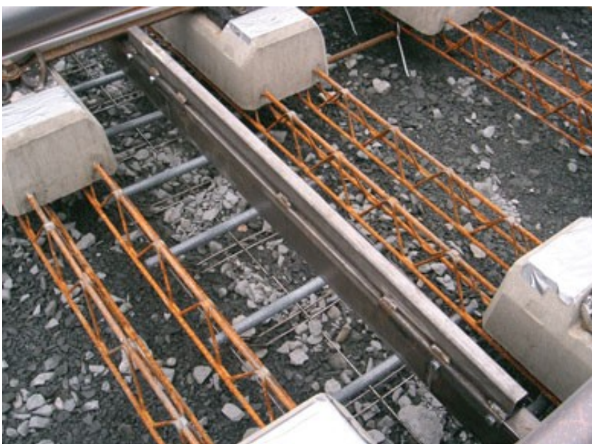
Figure 67 Rheda 2000 as installed, with controlled crack formation
