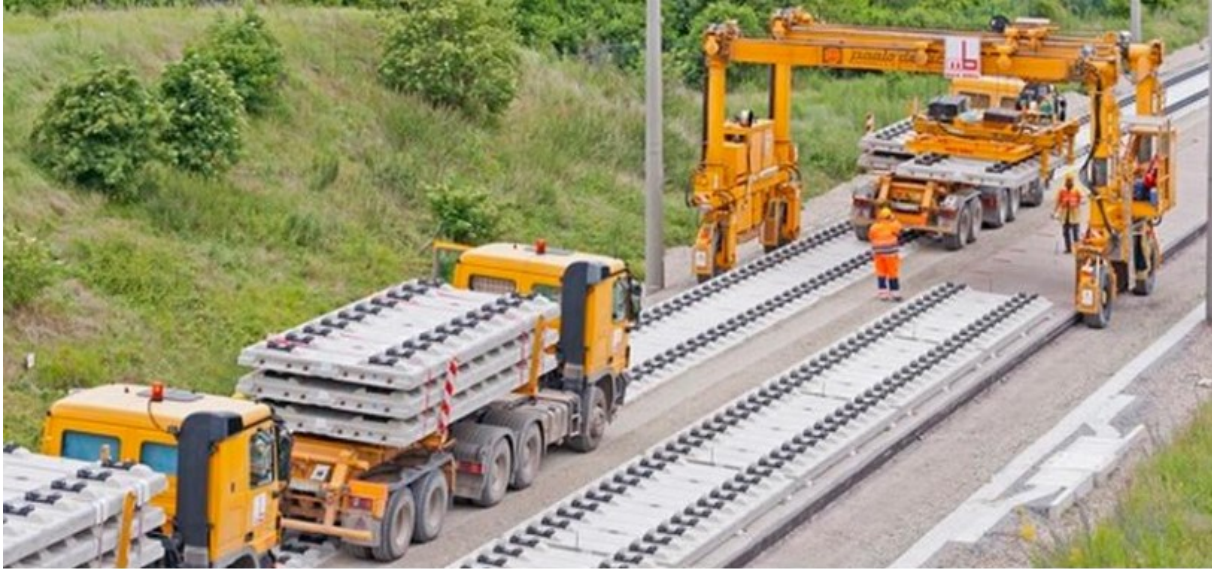
Figure 33 Transportation and rough placing of precast slabs, FFB Slab track Bögl (CEMOSA et al., 2014)
