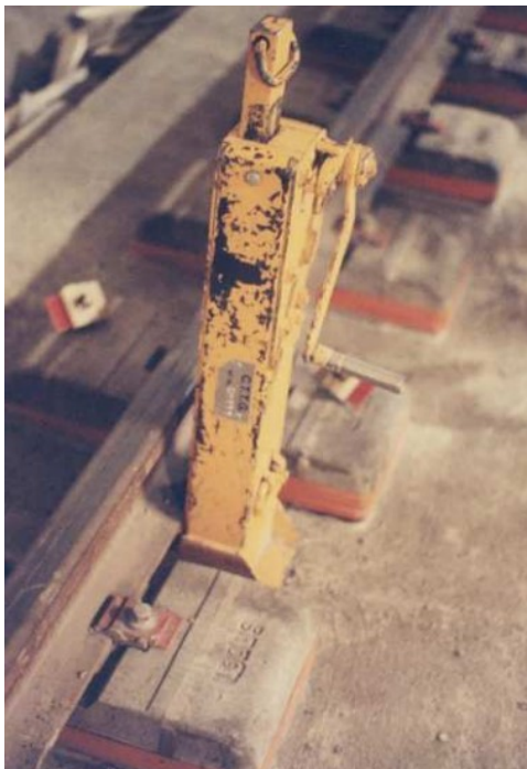
Figure 48 Lifting of rail LVT system (Sonneville AG, 2019a)
