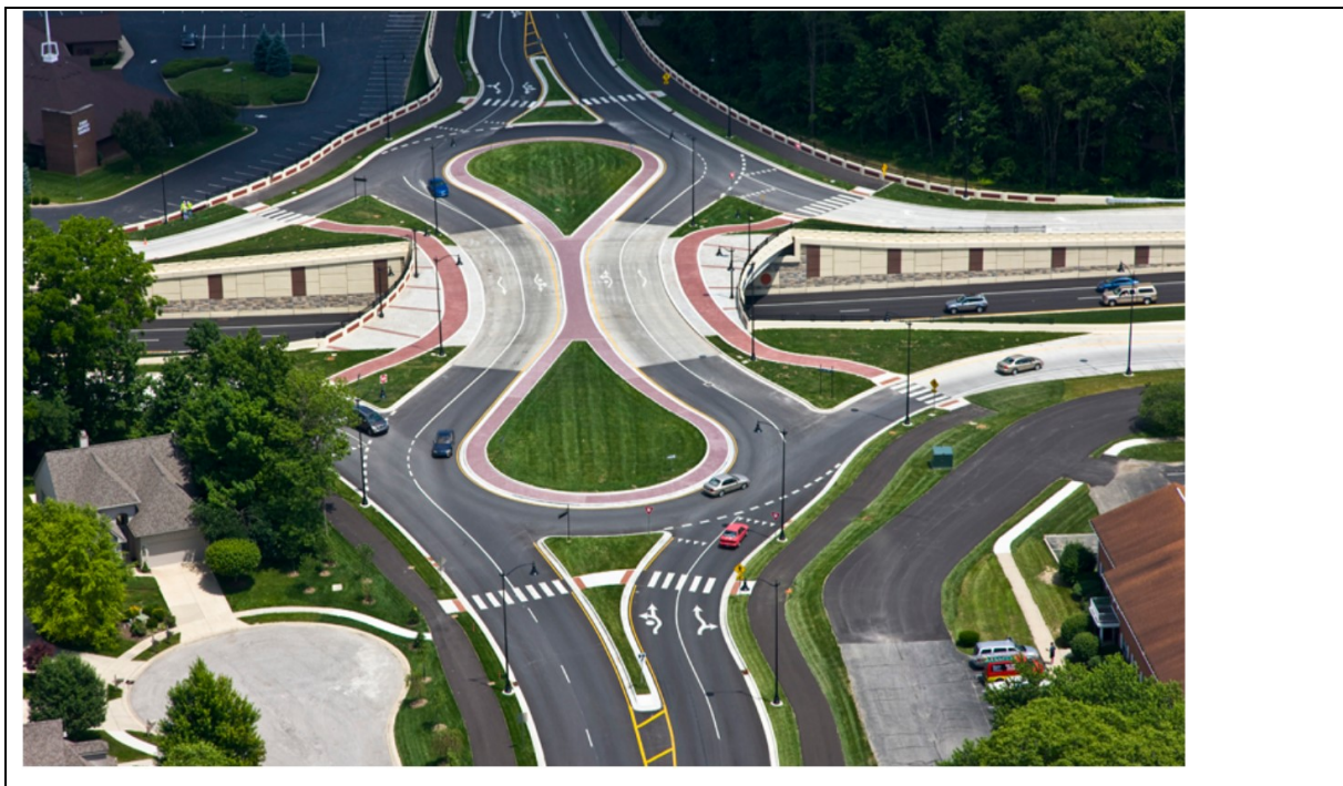
Figur 9: Dråperundkjøring i Carmel, Indiana, USA : FIGURKILDE: https://www.structurepoint.com/engineering-and-infrastructure/project/keystone-parkway-at-126th-street
