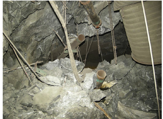
Fig. 5. A fault-slip rockburst triggered by a seismic event of M_n = 3.8 in a metal mine (Courtesy of David Counter).
