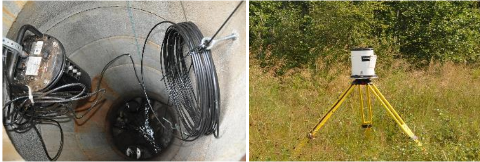
Figure 3.5 Flow meter (left) and rain gauge (right) in Lykkjebekken catchment.
