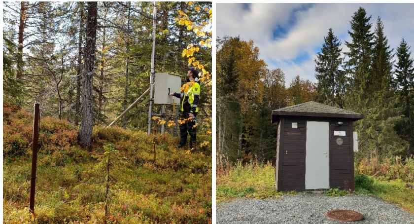
Figure 3.6 Groundwater well (left) and pumping station (right) in Lykkjebekken catchment.
