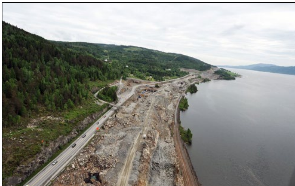
Figure 3.12. Embankment along Mjøsa due to establishment of roads and railroads.
