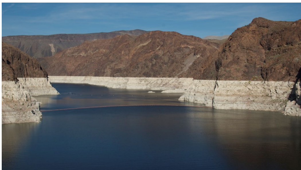
Figure 3.9. Lake Mead on Colorado River, dammed by the Hoover Dam, has been established in a canyon with a close to vertical shoreline, giving small dewatered areas when the water level drops.
