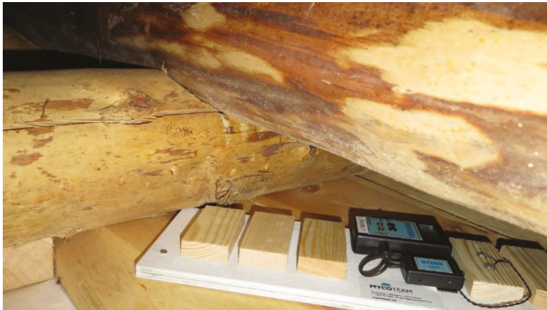
Figure 3. Climate panel. Photo: NIKU.
