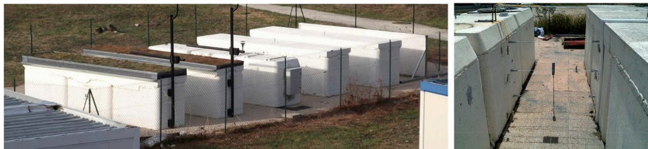
Fig. 7. Experimental facility in La Rochelle: the five rows of empty tanks simulating four canyon environments and view of the sensors installed in the canyon median.
