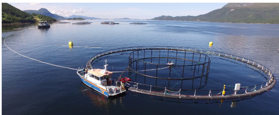
Fig. 2. The experiment cage, i.e. the floating collar along with the centered circular bird net frame (hamster wheel) is shown in the foreground. Also the feed barge can be seen in the background (top-left corner), as well as the white feed pipe running between the barge and the cage.
