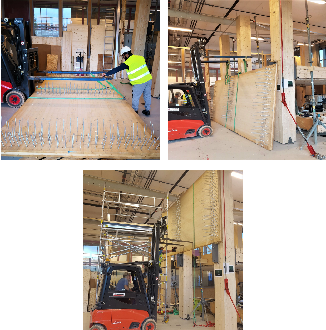
Figure 4.5: Installation of CLT to columns
