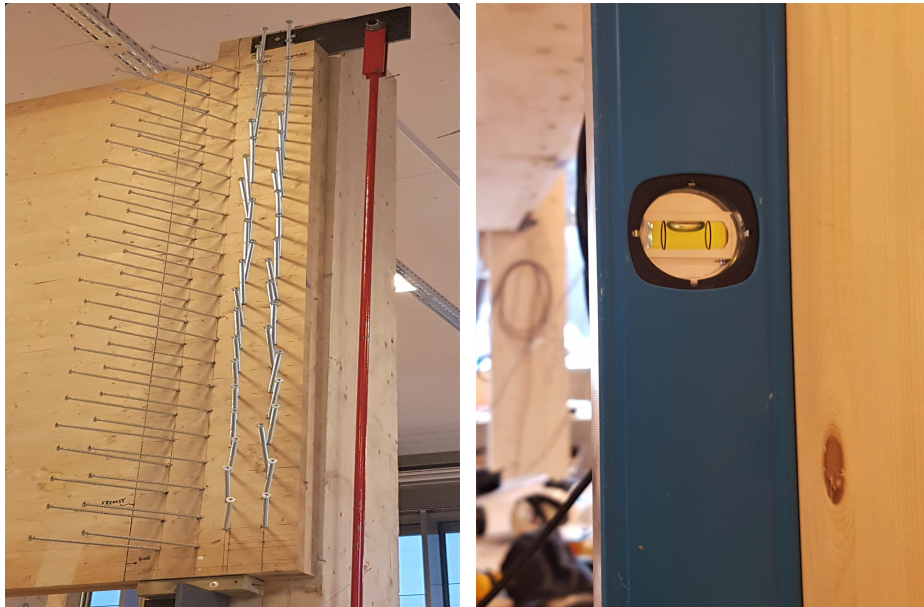
(a) Slightly misaligned column after Configuration 0
