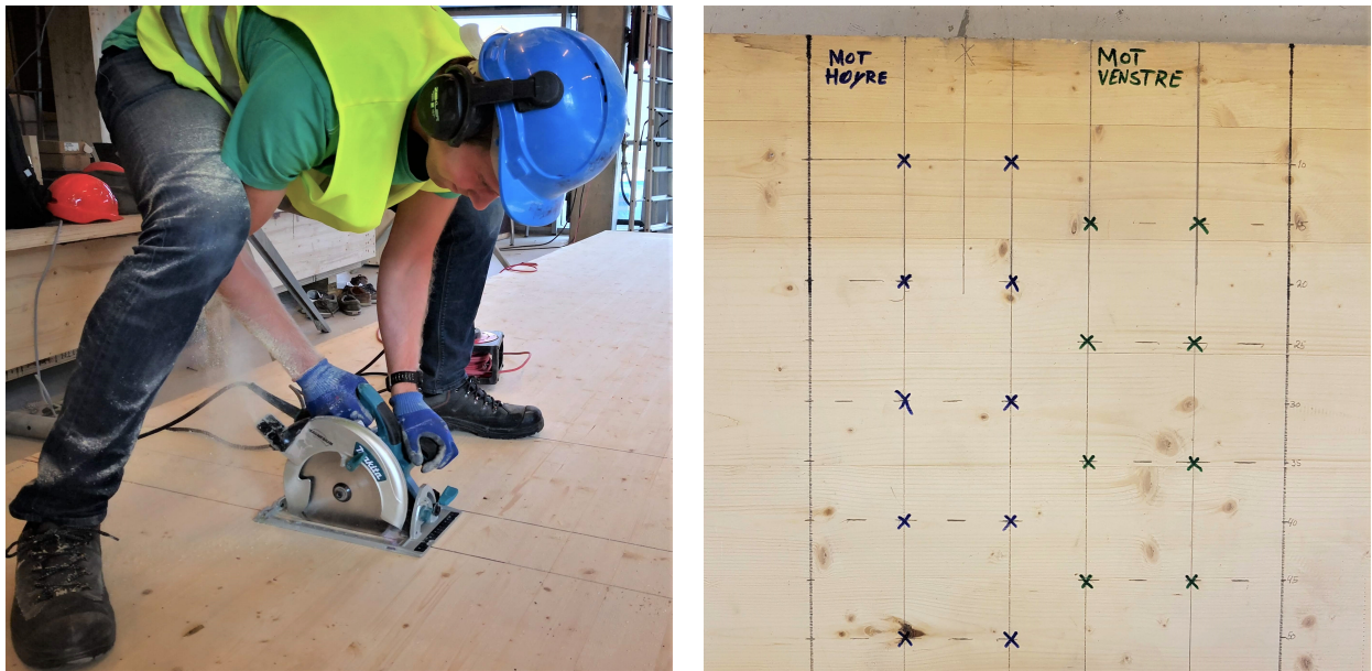
Figure 4.2: Adjustment and marking of the CLT panel
