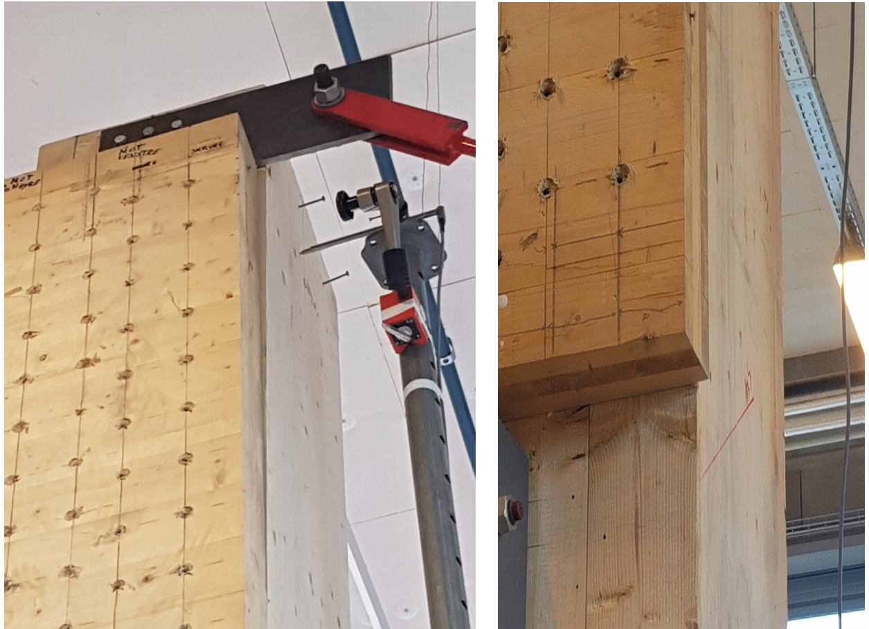
Figure 4.18: Slip between CLT- wall and column after tests on Configuration 9
