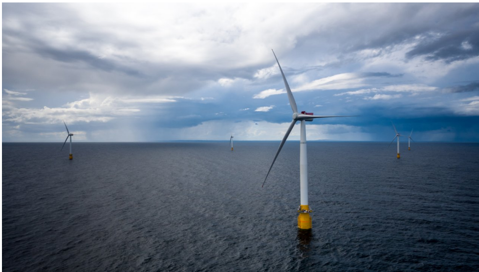
Figure 1.2: The Hywind Scotland floating wind farm by Equinor [6].
