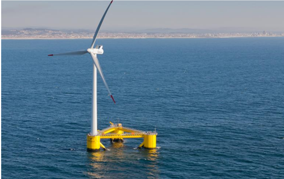
Figure 1.3: The WindFloat concept by Principle Power [9].
