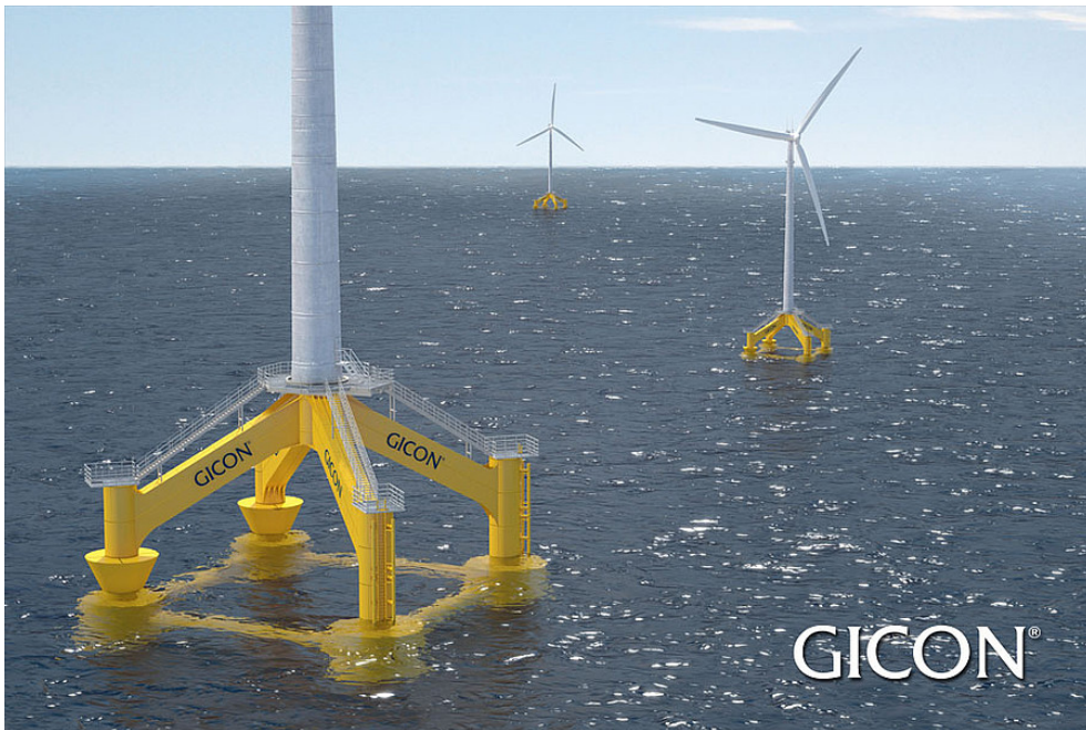
Figure 1.5: An illustration of the TLP concept by Gicon [12].
