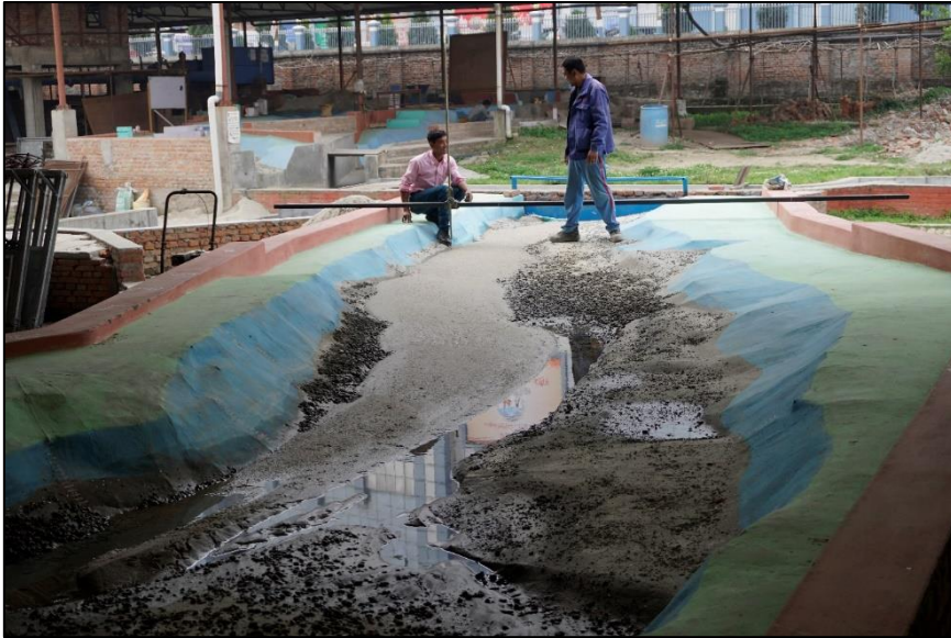
Figure 3-7 Manual cross-section measurement (Hydro Lab)
