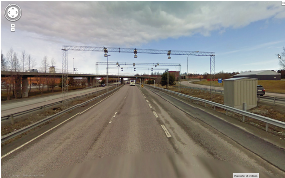
Figure 5.1: Toll Plaza near Kroppan Bru. Not necessarily room for stopping cars. Image attribution: Google Maps [19]
