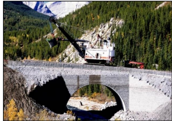
Figure 1.8 - Passage of 1144 tonn mining vehicle over the 24 meter long Whitehorse creek bridge (Bakht. B, 2007)
