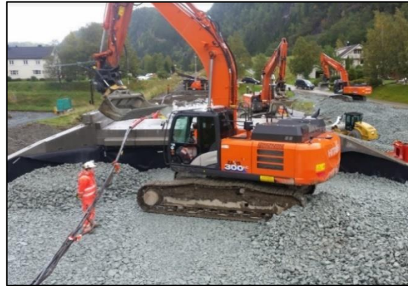
Figure 2.36 – Demonstration: Backfilling at Kilnes culvert from 2016, indicating that the material may be expected to be very rigid in relation to the culvert (FOTO: Farbu & Gausen AS)
