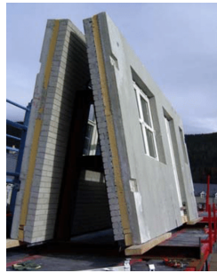
Figure 4.4: Prefabricated wall panel (ResearchGate, 2019)
