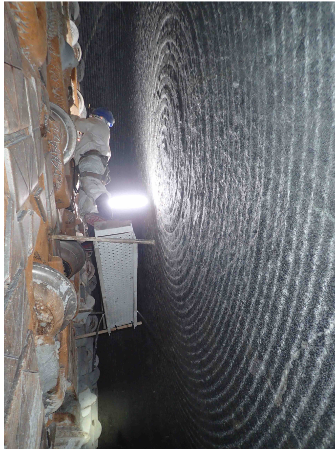
Figure 3.6: Kerfs a on stable working face at the Follo Line (Bane NOR)
