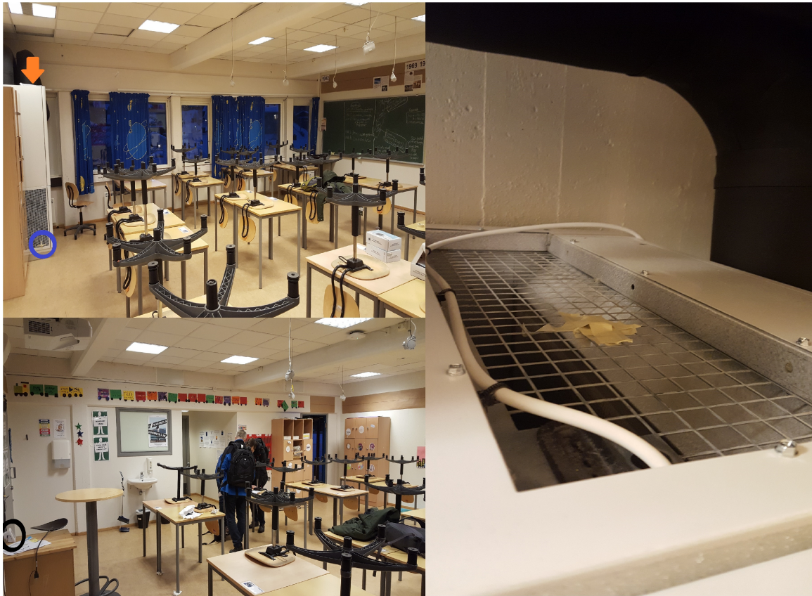
Figure 7: Pictures from Room 104. The supply air iButton is marked by a blue circle in the top left picture, the extract air iButton is indicated by an orange arrow. The ELMA monitor is marked by a black circle in the bottom left picture.
