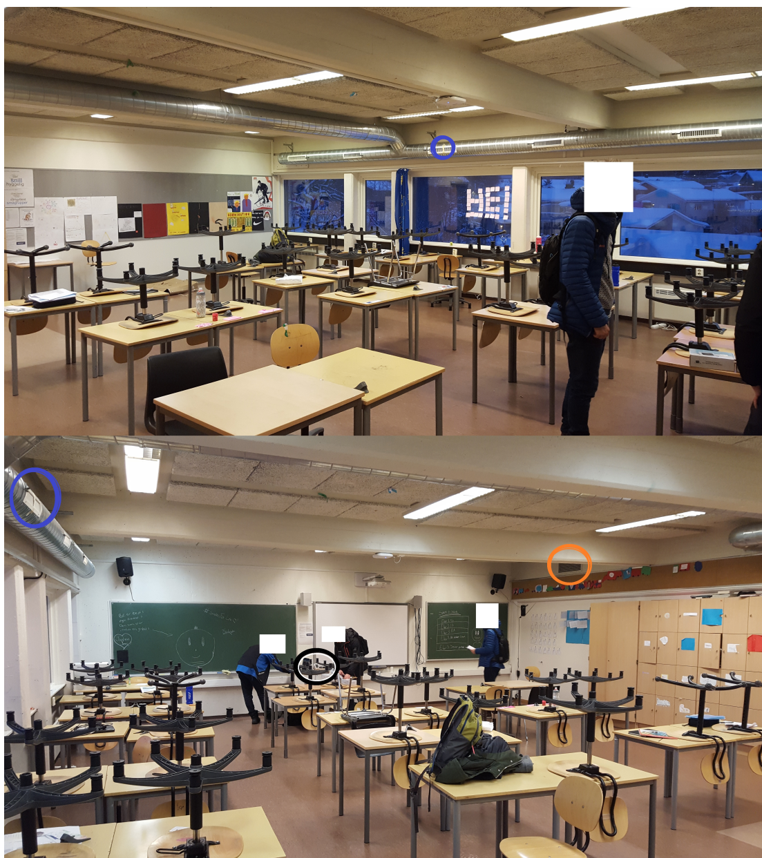
Figure 8: Pictures from Room 108. The supply air iButton is marked by a blue circle on both pictures, the extract air iButton is indicated by an orange circle and the ELMA monitor by a black circle on the bottom picture.
