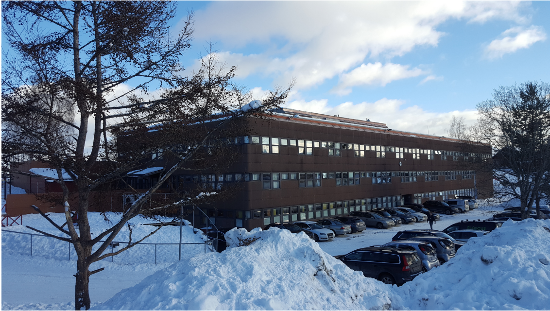
Figure 3: Picture taken from the northwestern side of Stabbursmoen school.
