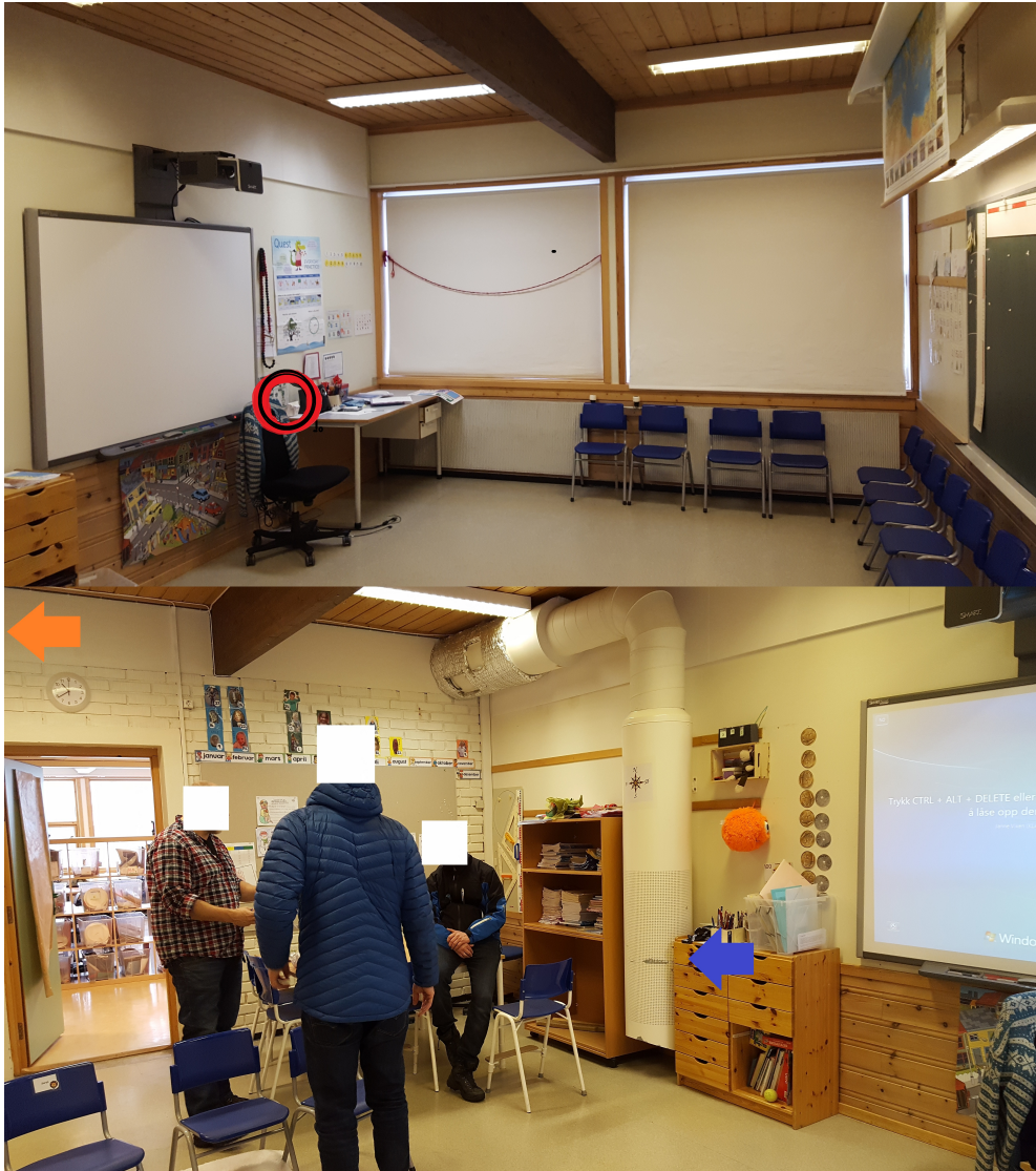
Figure 18: Pictures from Room 0273. The extract vent is not visible, but is located to the right of the door close to the ceiling. The ELMA monitors placement is shown by the red and black circle. The supply and extract air arrows placement are indicated by a blue and an orange arrow respectively.
