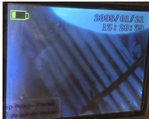
Figure 5.5: The exhaust outlet seen further away
