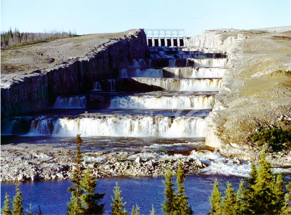
Figure 4: James Bay LG-2 spillway (Impregilo 2019)
