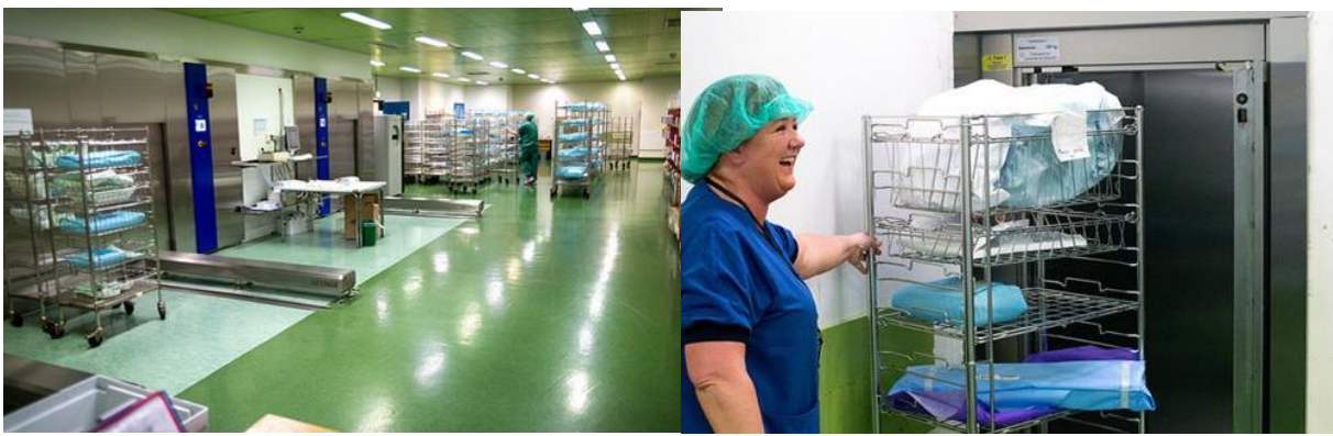
Figure 22: Unloading of Autoclaves, Sterile Storage and Clean Elevator (StavangerHF, 2016)
