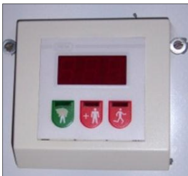
Figure A.5: Three button panel used in some isolation rooms (Kristiansen 2010b).
