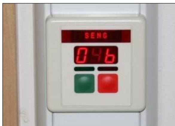
Figure A.2: Presence panel on the door frame (Kristiansen 2010a).
