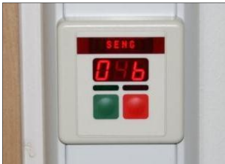
Figure 3.4: Presence panel located on the door frame of every patient's room (Kristiansen 2010a).
