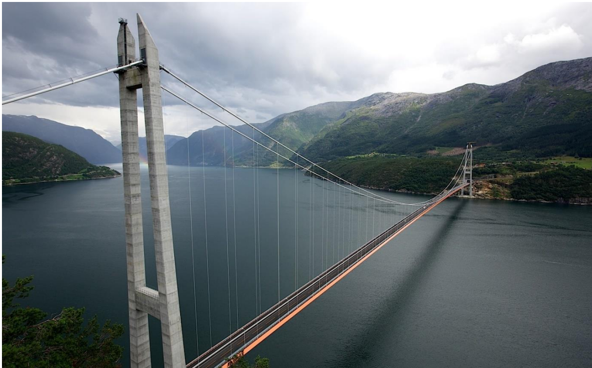
Figure 1.1 - Hardanger bridge top view (2)
