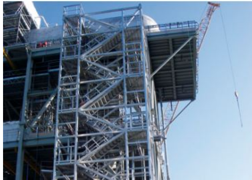
Figure 3.20: Aluminium stair tower for offshore installations.
