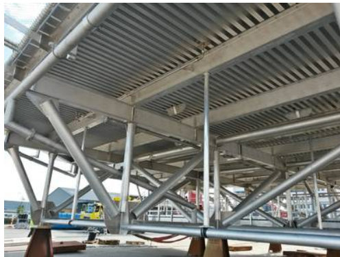
Figure 3.19: Aluminium profiles in a helideck made by Kapp Aluminium.
