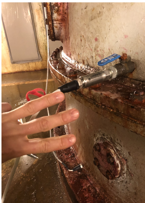
Figure 10.5: Picture of pressure transducer placed on the draft tube of turbine 3.
