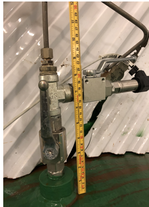
Figure 10.7: Picture of pressure transducer placed upstream the bulb valve, (PU1, PU2, PU3, PU4). The mounting is similar on all the turbines.
