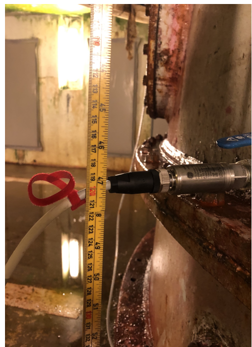
Figure 10.5: Picture of pressure transducer placed on the draft tube of turbine 3.
