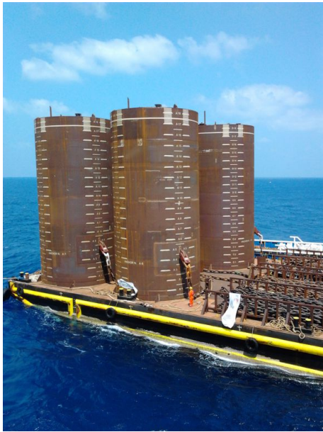
(a) Suction anchors (SPT Offshore, 2019)
