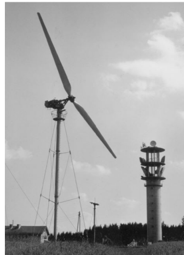
Figure 2.1.1: "Wind turbine by U. Hütter in Stötten in the Swabian Alb, Germany (rotor diameter 34 m, rated power 100 kW), 1958-1968", Hau (2013)
