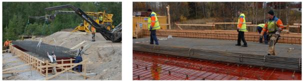
Figure 7: Use of prefabricated reinforcement cages (left) and rebar carpets (right).
