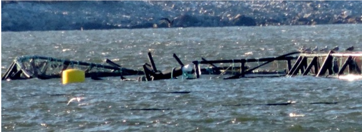
Figure 1.1: An example of structure failure
