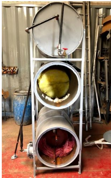
Figure 12: System during insulation process
