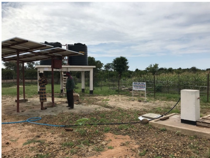
Figure 9.5: Solar powered pumping system, both clean and with a good fencing system.
