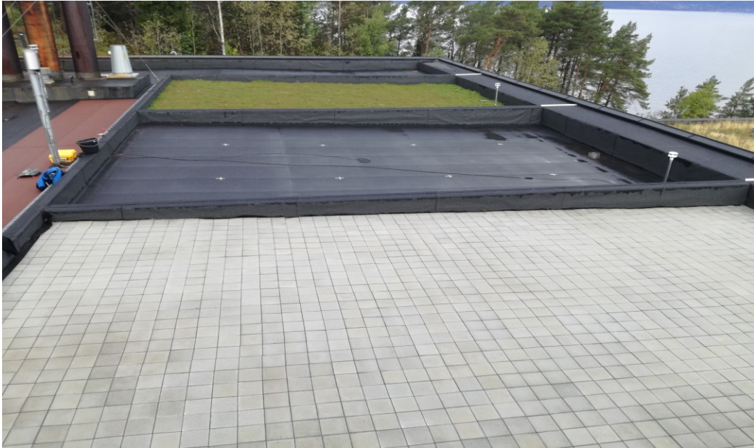
Figure 2.2. A full-scale view of the pilot grey roof (closest) together with black conventional (reference) roof (middle) and green roof (furthest).
