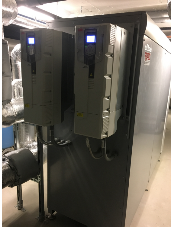
Figure 2.8: Picture taken by Mathias Metlid in September 2018 of the heat pump unit
